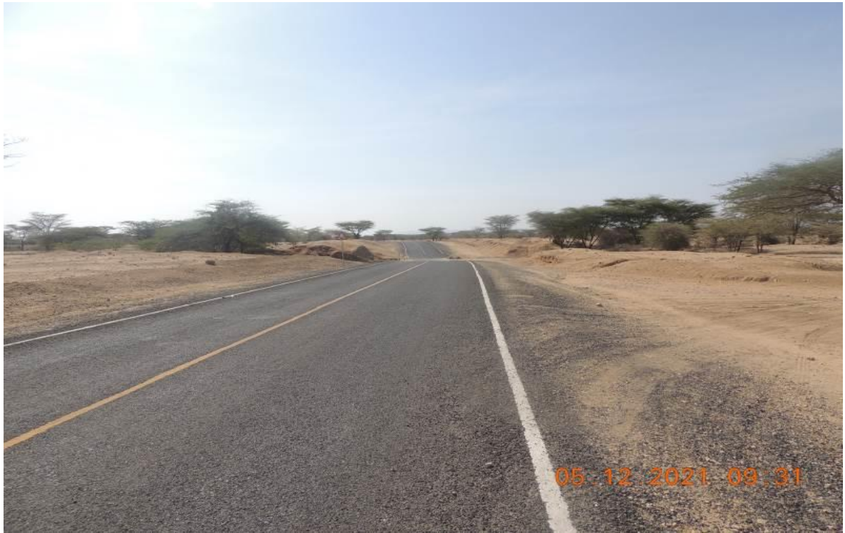
Plate 2-8: Pipeline Crossing Point Across C46 Road
