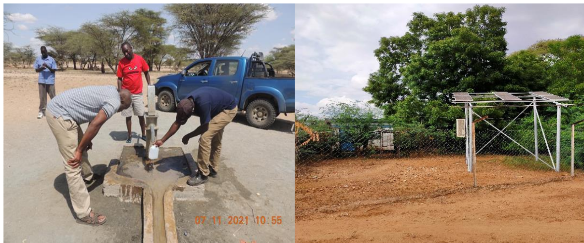
Plate 5-10: Groundwater abstraction in the project area. Left: Shallow well at Kamarese; Right: Solar powered 98 m deep borehole at Nakwamoru.
