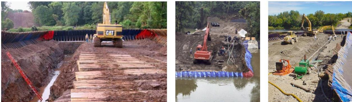
Figure 2-11: Open Cut River Crossing Using Portadam
