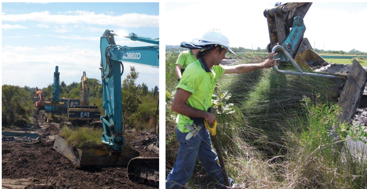
Figure 1 Systematic placing of whole turves using modified machinery. (Photos: Stocklands Bundilla)
