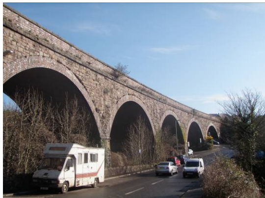
Figure 4.4: Viaduct with medium height piers
