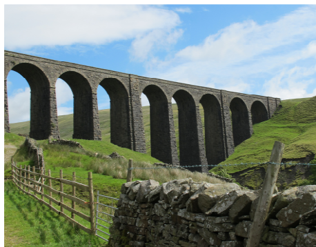
Figure 4.2: Slender multi span viaduct, Arten Gill, Cumbria
