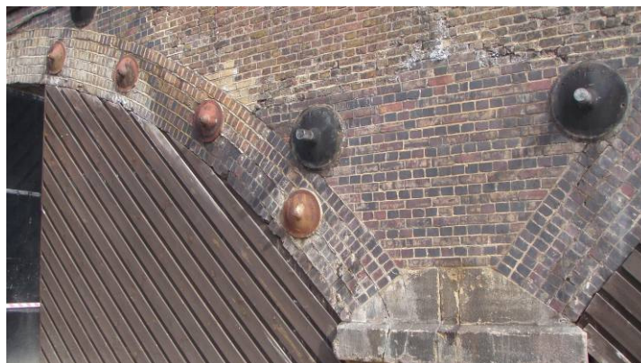
Figure 4.6: Extensive strengthening, Chelsea River Bridge northern approach
