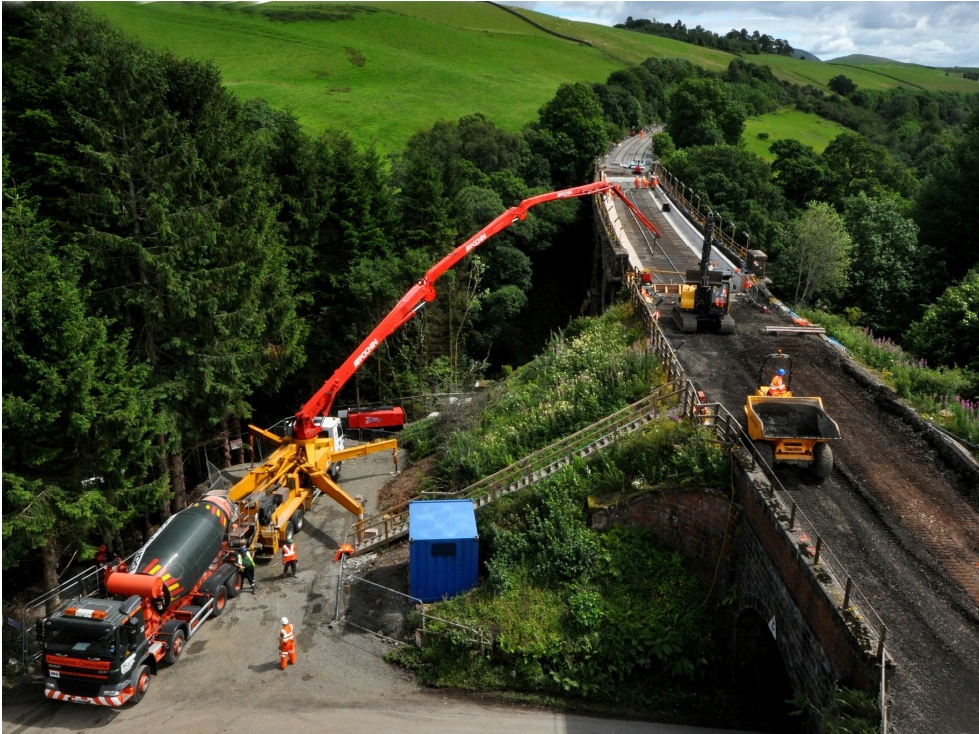
Figure 5.5: Construction of concrete saddle at Enterkin Burn, Scotland
