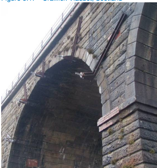
Figure 5.1: Crawick Viaduct, Scotland
