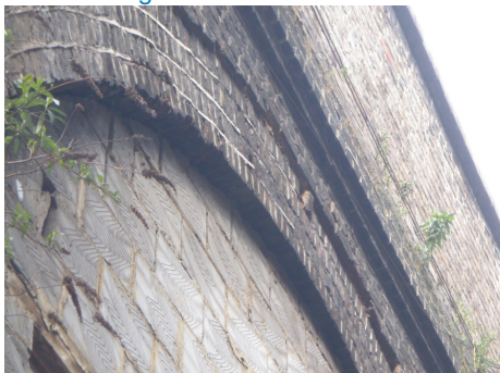
Figure 2.3: Sliding failure
