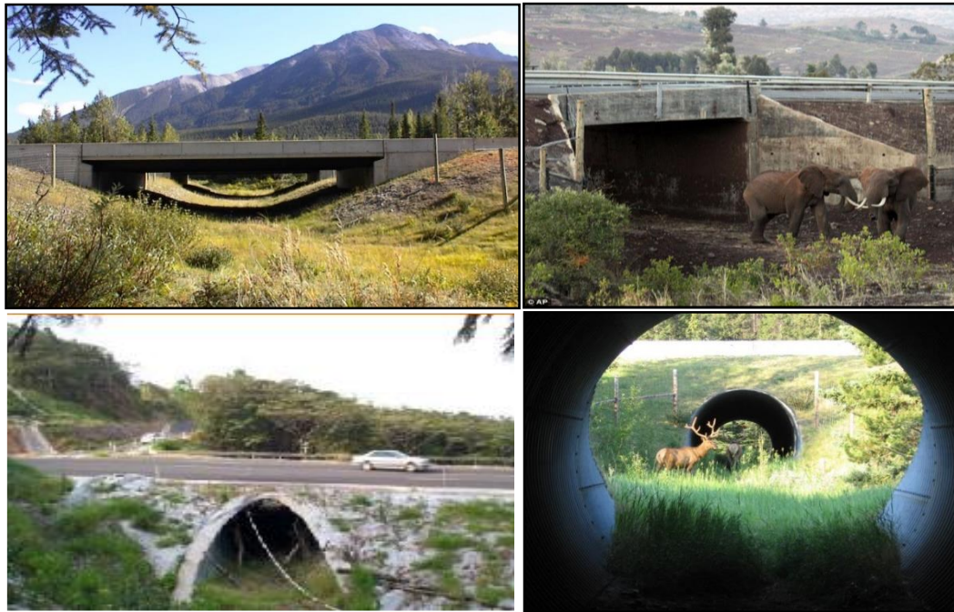
Figure 5.2: Bridge underpasses and culverts designed to facilitate animal movement
