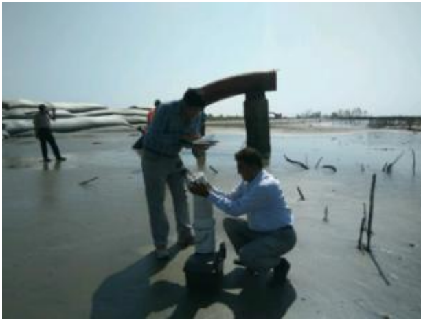
Picture 7: Air monitoring near the EEBL FSRU Tie-in-Point.
