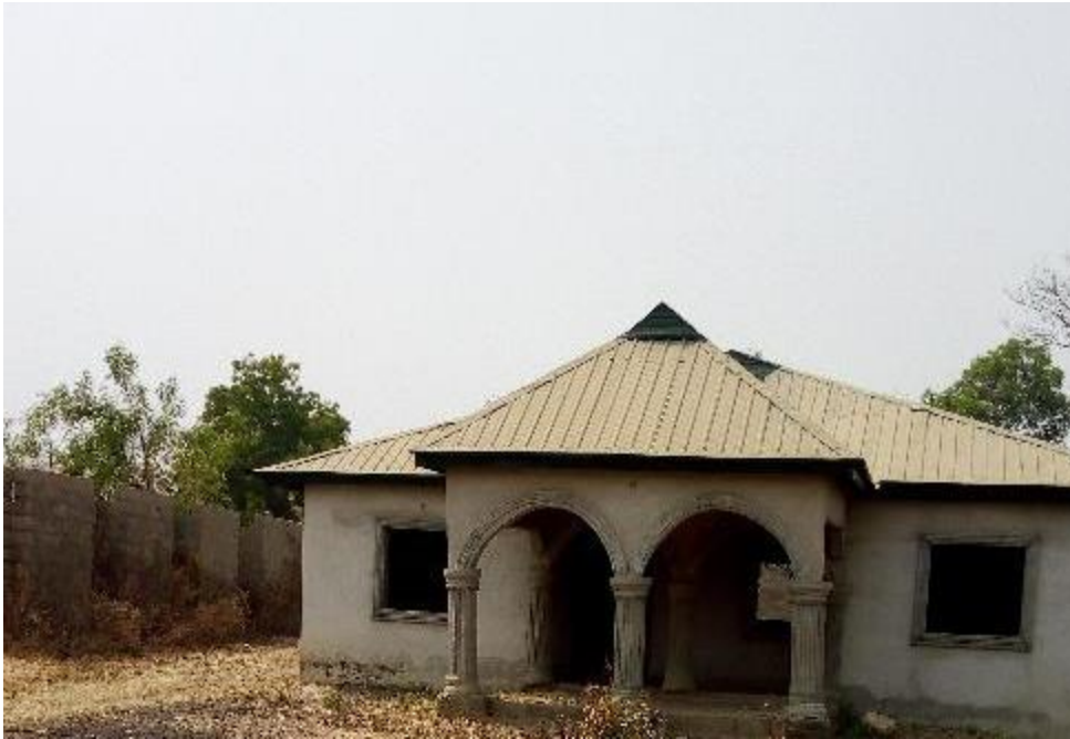
Plate 4.10b: A modern house under construction observed in Ajaokuta
