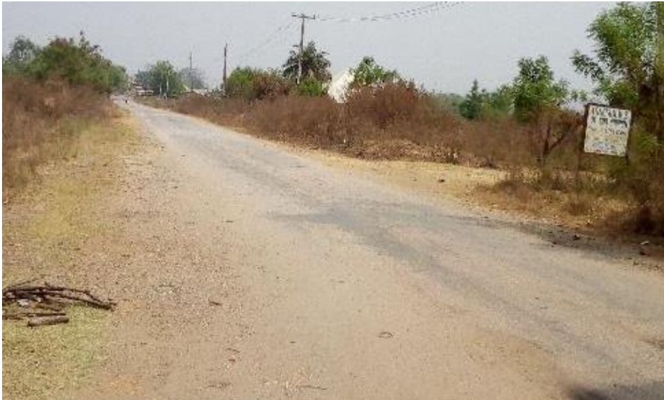
Plate 4.13a: Section of the main road leading to Ajaokuta
