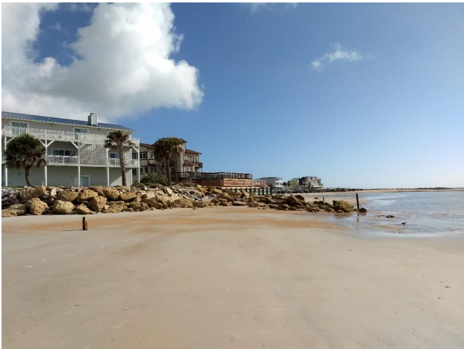
Figure CS3-7. Significant beach erosion has occurred at Vilano Point due to the recent hurricanes and Nor'easters. County staff indicated that prior to 2017 the rock berm shown here was entirely covered by sand.
