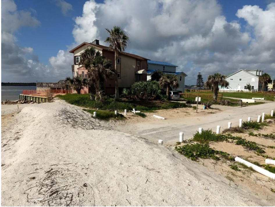
Figure CS3-6. A temporary sand berm has been placed at the end of a street in Porpoise Point. During recent storms, storm surge overwashed the beach and funneled into the subdivision at this location.
