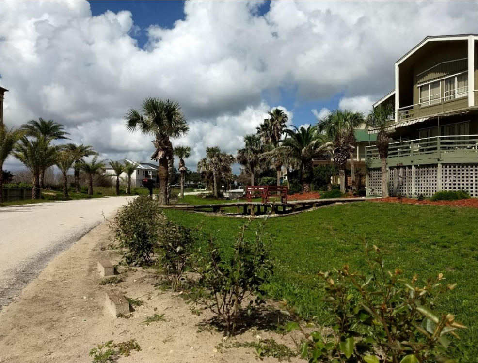
Figure CS3-9. Example of current stormwater swales at Porpoise Point.
