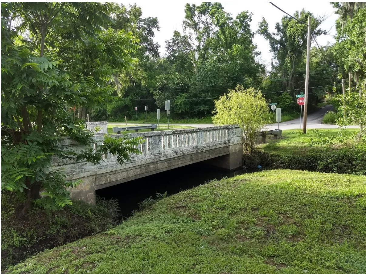
Figure CS1-6. McCoy Creek Boulevard at Hollybrook Park, an area subject to frequent flooding. Several low-grade bridges like the one shown restrict the stream channel and three are targeted for replacement.
