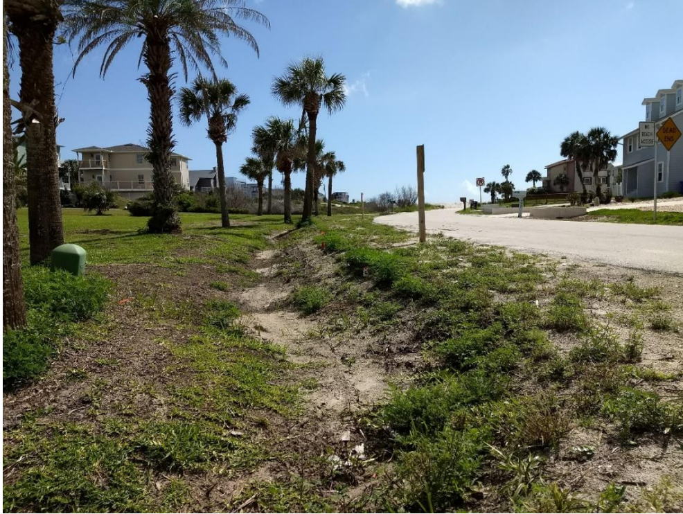
Figure CS3-8. Example of current stormwater swales at Porpoise Point.
