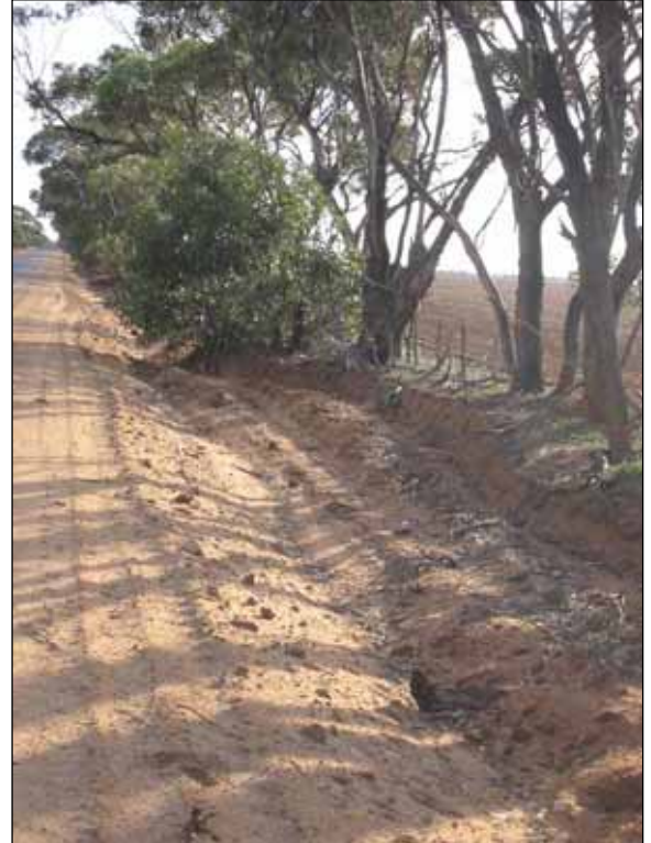
Regular road maintenance should avoid the root zone of adjacent native vegetation where possible.
