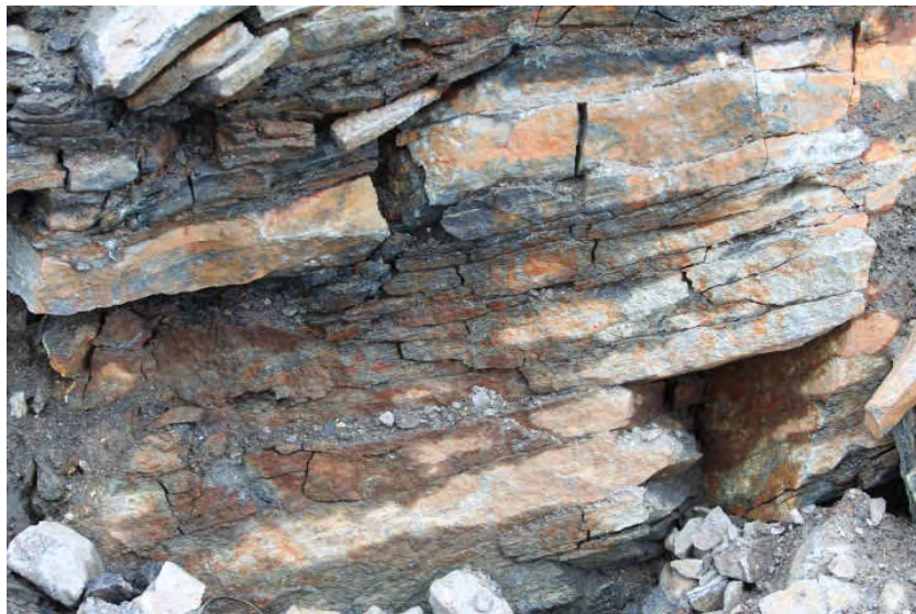
Figure 5.25 The bedrock of foundation site No. 2.8 in the Mehuken II windmill park consists of augen gneiss and amphibolites (Photo: Ragnar Hagen). The 21.6 m-long core indicates competent bedrock, except for a few zones where the drillcore is very heavily fractured or totally crushed (Göthfors 2010 and Appendix 2). These fracture zones contain an abundance of clay minerals. Otherwise there are very few fillings in the fractures. Fracture minerals present are clay minerals and chlorite. See Appendix 2 for further details.
