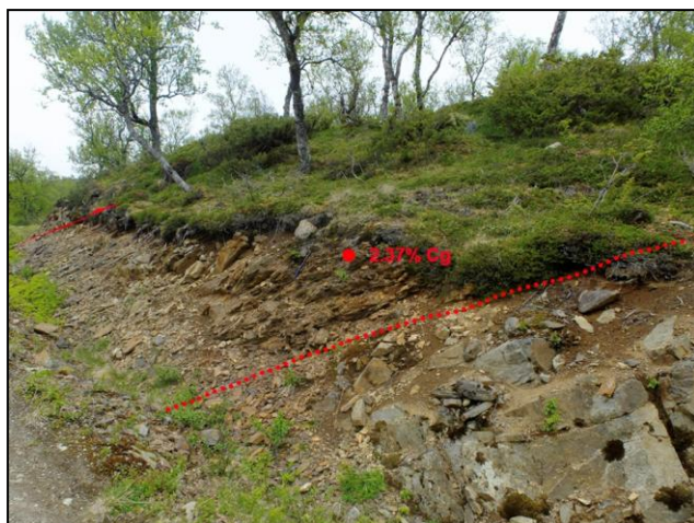
Figure 18. Road-cut at Koven with exposed graphite mineralisation and % Cg in a sample collected.
