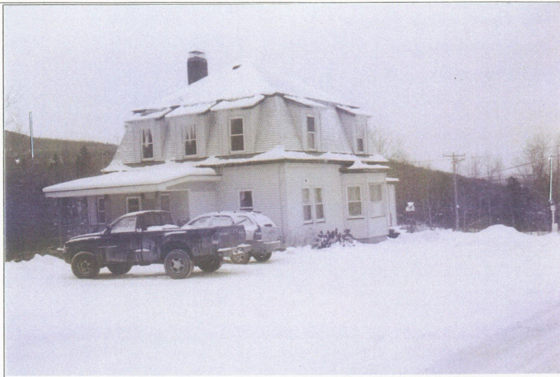
Photo 21 description: The Balsams Worker Housing – 12 Trailer Road Property, House Roll: 3 Frame: 5 Direction: Southwest Date taken: December 2007 Negative stored: NHDHR
