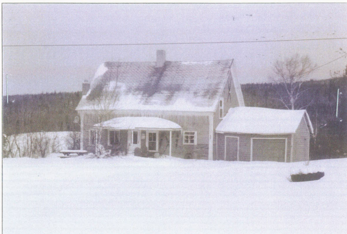
Photo 16 description: The Companga House, Front Facade
