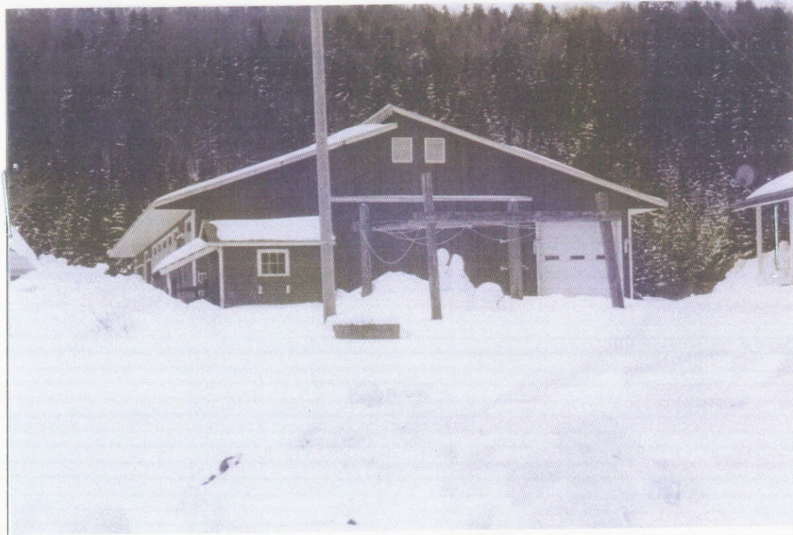
Photo 12 description: The Sweatt Farm, Pole Barn
