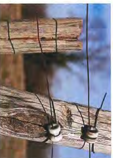
Electric fences are specially insulated from the ground and can pick up an induced charge from transmission lines.
