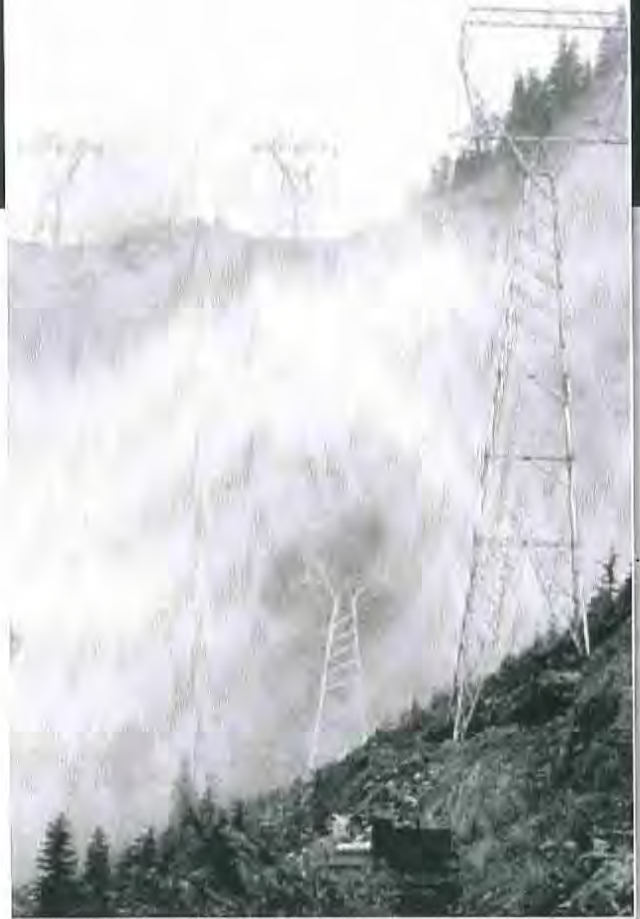
A fire burning under a power line can create a dangerous situation. Stay away from lines if a fire is nearby.
