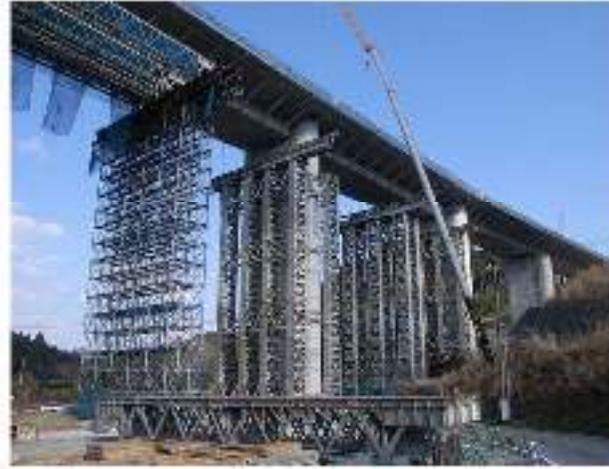
Launching method by using track and crane
