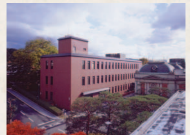
Conservation Center for Cultural Properties
