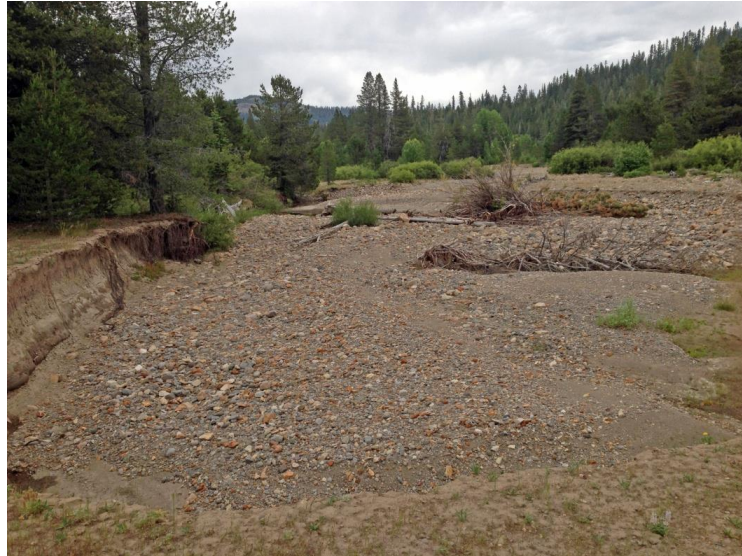
View of Middle Yuba River channel showing the cut bank, scour, and erosion resulting from frequent high flow events (Beedy 2018).
