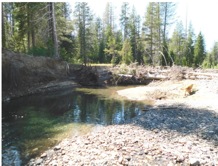
Middle Yuba River showing bank erosion and subsequent debris. (Neysa King, NID)
