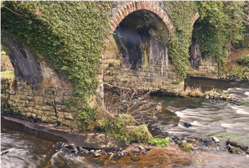
Moyola River, Old disused railway bridge. Photograph by Nigel Ready
