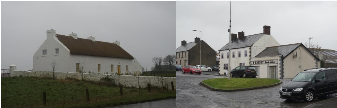
L-R Restored cottage near Bellaghy Bawn formerly on at risk register and renovated with a DfC grant and streetscape view adjacent to the Bawn. Photographs by Marianne O’Kane Boal
