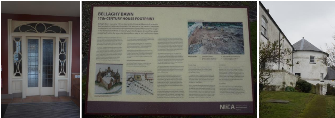
L-R Bellaghy Bawn Interior door and fanlight, sign for 17 th century house footprint and view of Bawn. Photographs by Marianne O’Kane Boal
