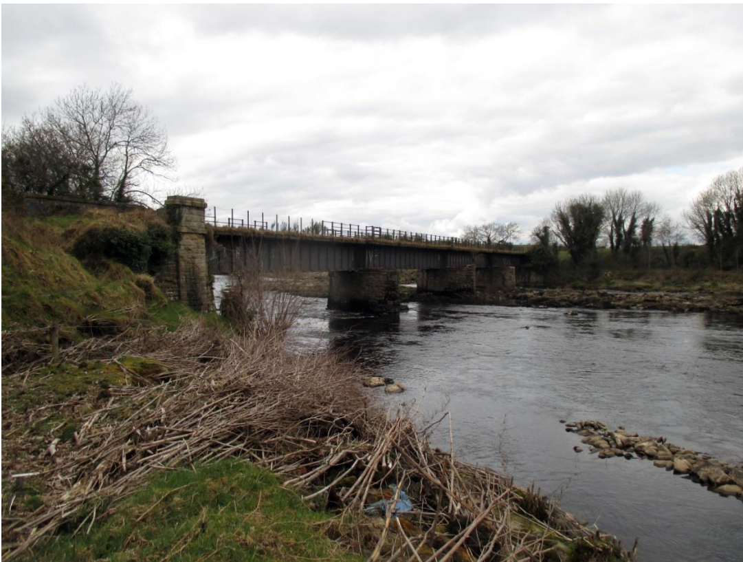
Victoria Bridge Camus metal railway bridge
