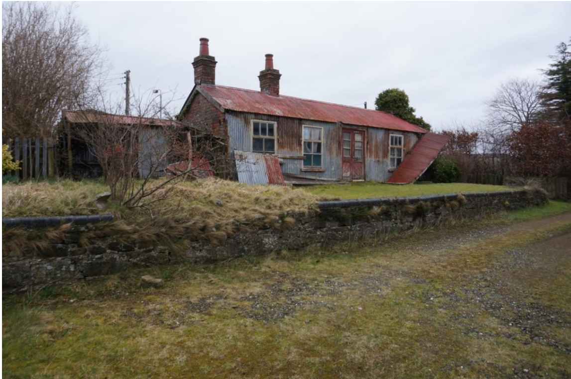
Ballymagorry Station and platform View 2
