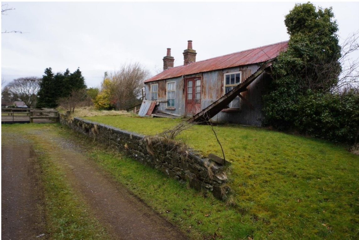
Ballymagorry Station and platform View 1
