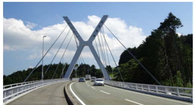
Photo: Kuwazuru Bridge after restoration
