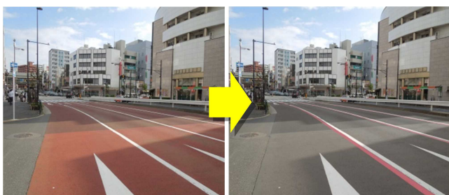
Fig. 1 Example of "Downsizing / Scaling down" Change from the whole surface colored pavement to line painting will reduce landscape obstruction and reduced area of painting on the spots where cars are unlikely to stop will reduce frequency of repair.
