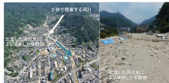
Photo 1: Sediment and flood inundation in the July 2018 Heavy Rain
