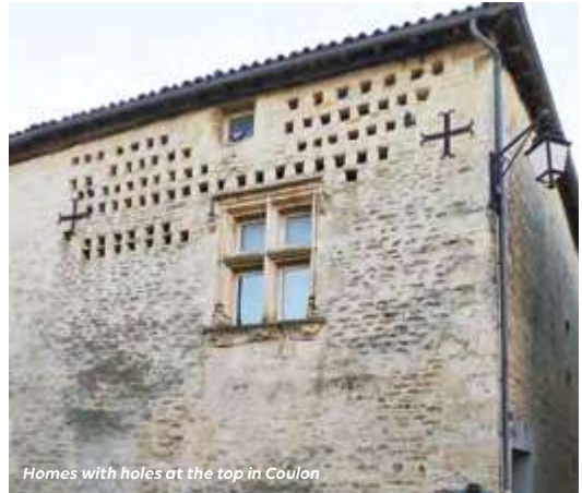
Homes with holes at the top in Coulon
