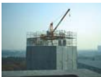
Self Jack-up & down tower crane
