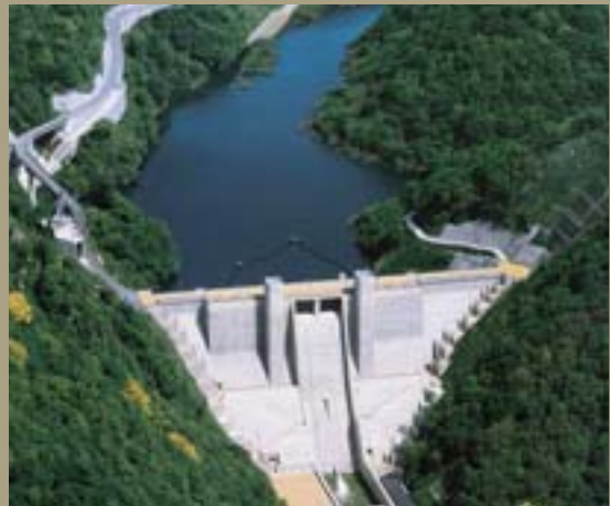
Ishii Concrete Gravity Dam
