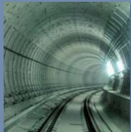
The Kaohsiung Metropolitan Mass Rapid Transit System, Red and Orange Lines, CR2 Construction Section, Taiwan
