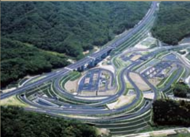
Seto-Akazu Interchange Construction, Tokai Ring Road
