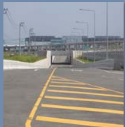
Airside Road Tunnel of Landside Road System, Second Bangkok International Airport, Thailand
