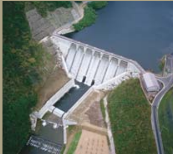
Masudagawa Concrete Gravity Dam
