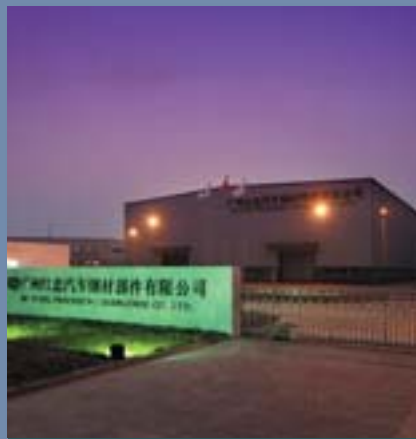
Marubeni-Itochu Steel Guangzhou Factory, China
