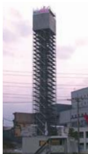
Erection of scaffolding for dismantling
