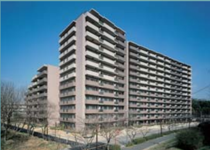
Laurel Coat Shin-senri Higashimachi Akashyanooka Residential Building
