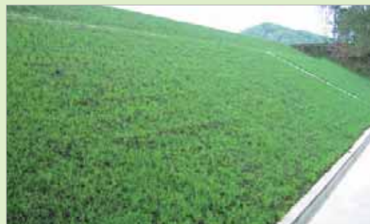
Completed Embankment Greening
