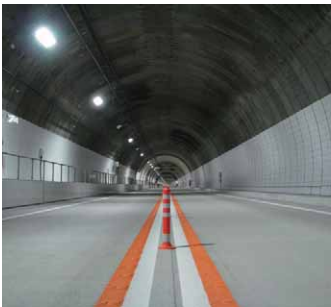
Hida Tunnel Phase 4, Tokai-Hokuriku Expressway
