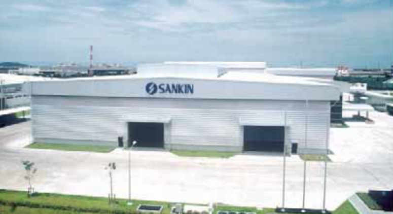
Sankin (Thailand) New Factory, Thailand
