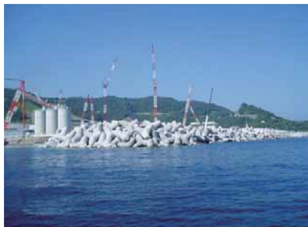
Breakwater Construction, Shimane Nuclear Power Plant
