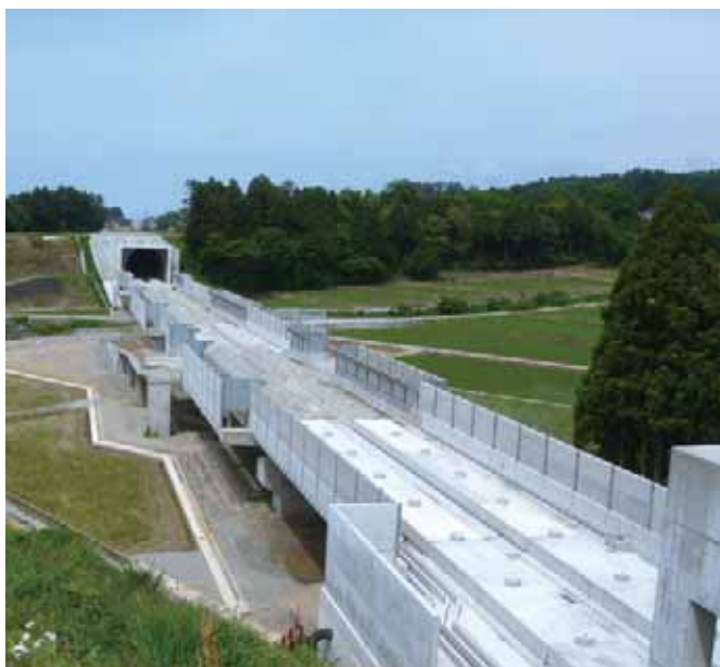
No. 1 Kurobe Tunnel, Hokuriku Shinkansen
