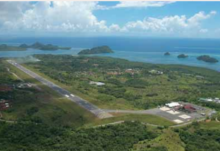
Palau International Airport Runway Resurfacing Project, Palau
