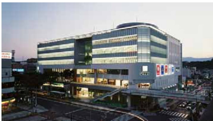
Mixed-Use Construction, Iwaki Station-Front First Class Urban Redevelopment Plan
