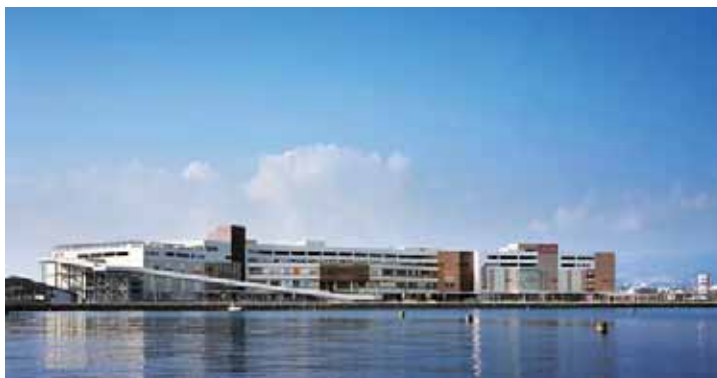
Aeon Kagoshima Tokaicho Shopping Center Construction
