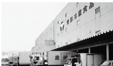
1980: Tobu Reizo Shokuhin's Hachioji Coldstore Hachioji City, Tokyo 10,064 tons
