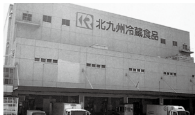
1986: Kitakyushu Reizo Shokuhin Coldstore Kokurakita Ward, Kitakyushu City, Fukuoka Prefecture 12,116 tons
