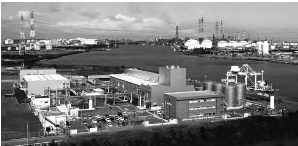
The Kashima Plant: The second construction phase was completed in October 2008.
