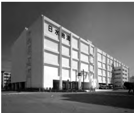
Nissui Logistics Corporation Kawasaki Distribution Center
