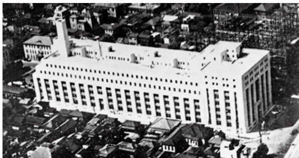
The Nissan Building Nippon Suisan moved its Head Office here from the Maru Building in August 1937.
