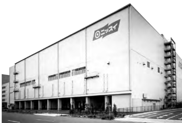
Tokyo General Logistics Center
