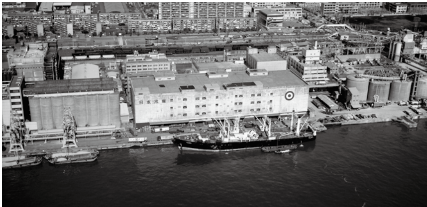
Harumi Coldstore (bird's-eye view)
