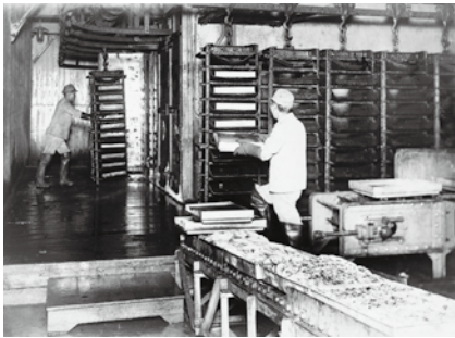
Work in progress in the rapid freezing room
