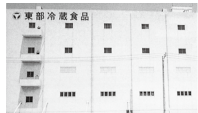
1987: Tobu Reizo Shokuhin's Funabashi Coldstore Funabashi City, Chiba Prefecture 12,430 tons
