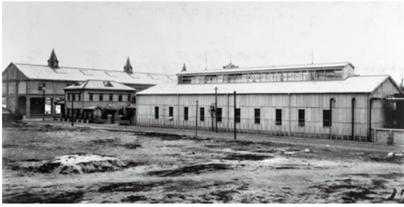
From the right: Machine room, office, pump room and landing yard. In the foreground, the site scheduled for construction of Tobata Seikan.
