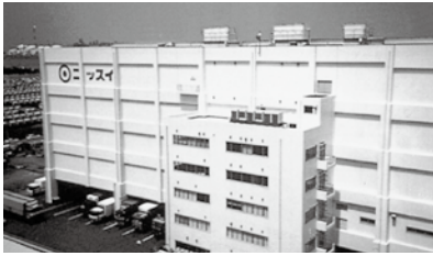
1990: Nippon Suisan's Kawasaki Coldstore Kawasaki Ward, Kawasaki City, Kanagawa Prefecture 31,200 tons
