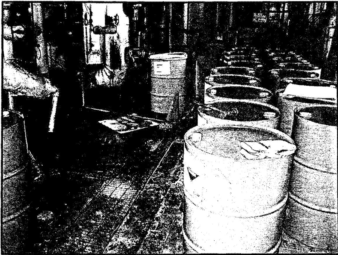
A chemical storage area and floor trench inside Building #28, built as brick floor.
