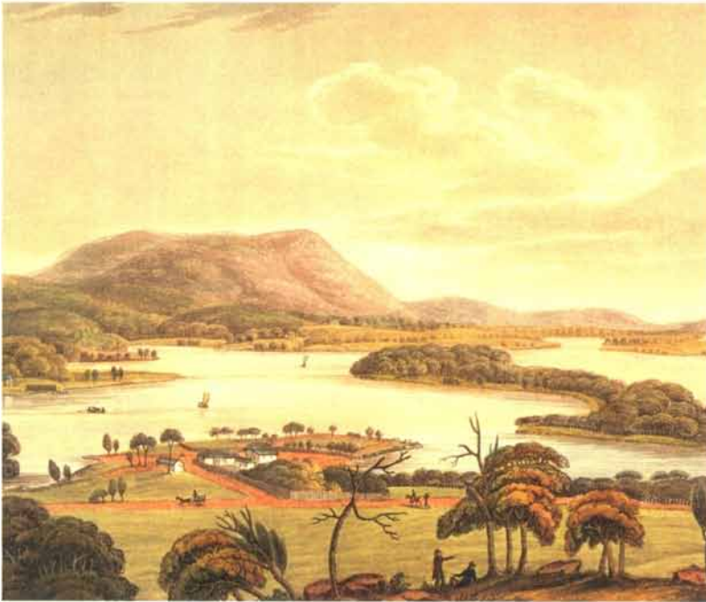
Cleared landscape and fenced garden of an early settlement near Hobart
