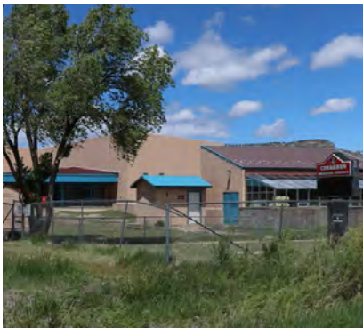
Damaged fencing and lack of security at Cimarron School Campus.
