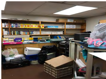
Eagle Nest School storage – poor location and usage for school needs.
