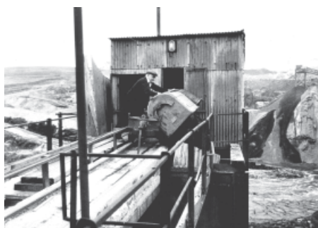
PLATE 24. Tipping trams, Whiteheaps Drift. (Courtesy H.M. Parker ©, 1973).
