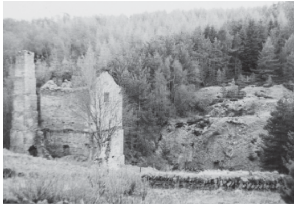
PLATE 27. Shildon engine house, view looking west from Shildon Lane, (1980).
