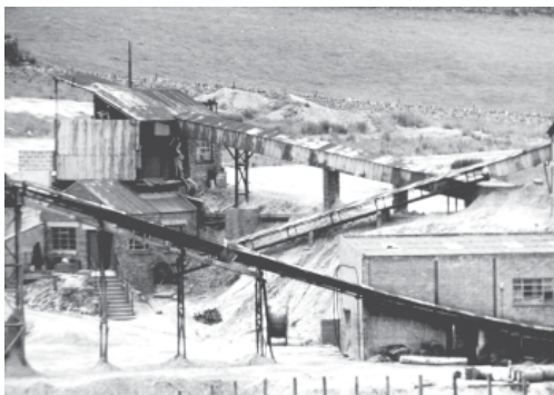
PLATE 25. Part of dressing plant, Whiteheaps Mine, pre-BSC (1981).
