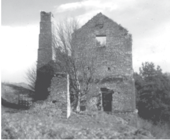
PLATE 8. The existing northern style engine house at Shildon Mine (1967).
