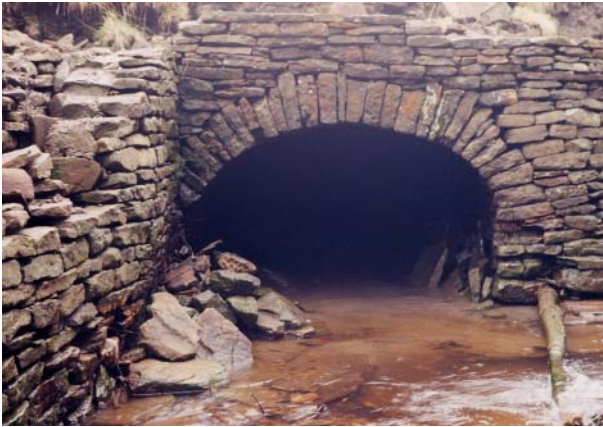
PLATE 49. Outfall of Bolts Burn from below Deborah dressing floor (1999).
