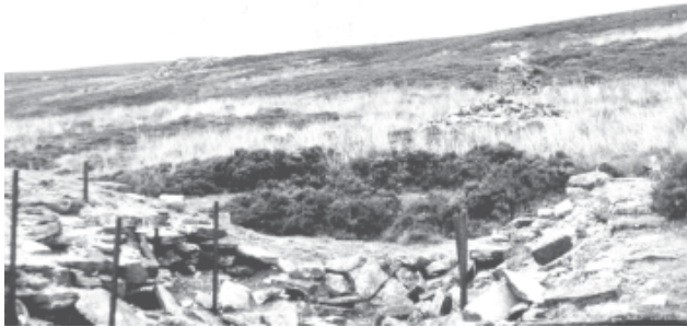
PLATE 10. Piers supplying water to engine at Westgarth's Shaft, Jeffreys Rake (1980).
