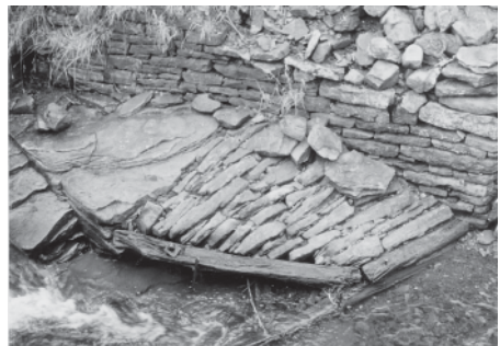
PLATE 50. Stream channel protection, Bolt's Burn (1999).
