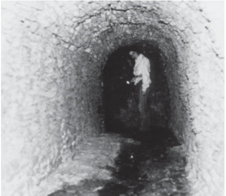
PLATE 46. Inside flue, Derwent Smelt Mill (1980).
