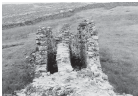
PLATE 54. Close view of condenser. Note horizontal flue track, and square chimney, top left, on horizon (1980).
