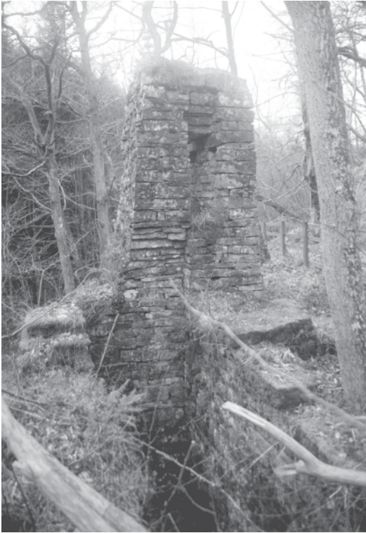
PLATE 42. Hisehope shaft wheelpit and beam support pillar (1999).
