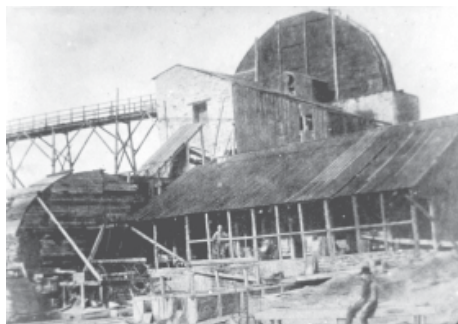
PLATE 37. Healeyfield Mine dressing floor (c.1880's, courtesy J. Raine).
