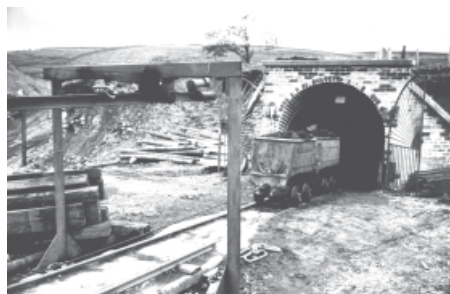
PLATE 23. Tram road, Whiteheaps. (Courtesy H.M. Parker ©, 1973).
