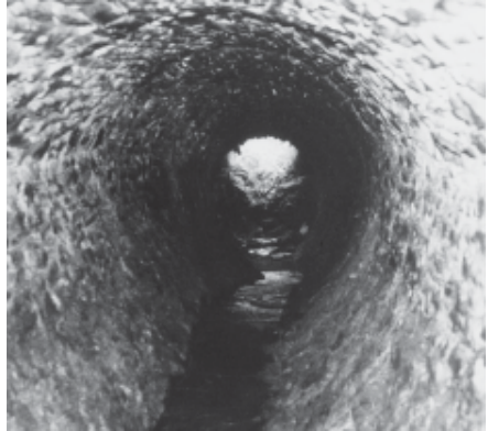
PLATE 47. Inside barrel flue, Derwent Smelt Mill (1980).
