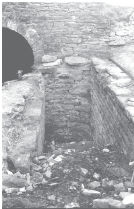
PLATE 4. Wheel pit and balance bob chamber at Ramshaw (1982).
