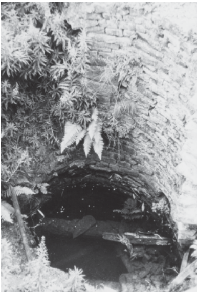
PLATE 33. Round pumping shaft, Beldon (1980).
