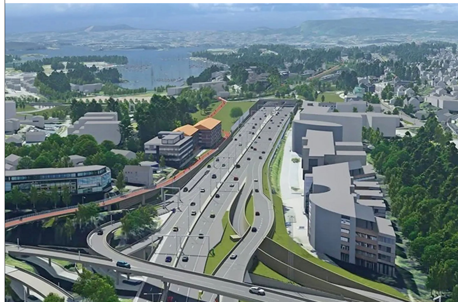
E102 – E18 highway Fornebu intersection to Strand (Statens Vegvesen/ViaNova)
