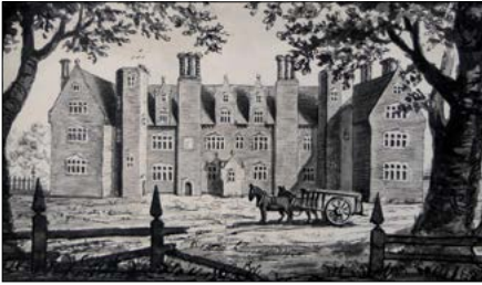
North side of Irmingland Hall nine years before most of it was demolished
