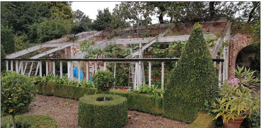
The old structure before demolition
