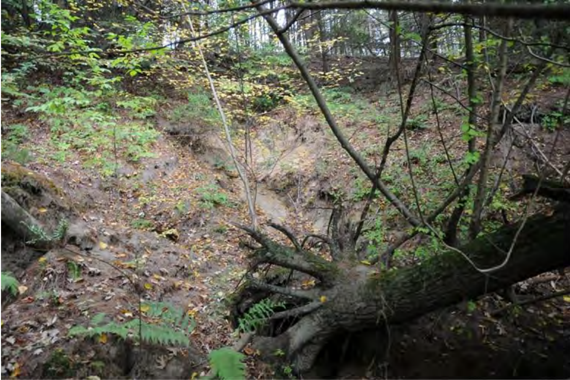
Figure C-12 Upland erosion feature (Photo 9517)
