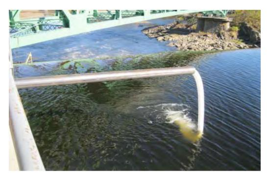
Figure 4-11 Metal pipe extension to release shad to the desired release point to ensure fish would pass over the Bascule Gates.
