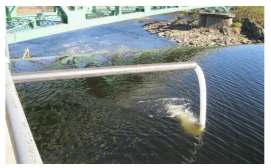
Figure 4-5: Six-inch diameter steel pipe with inserted four-inch diameter flexible hose that directed eels towards Bascule Gates 1 and 4.
