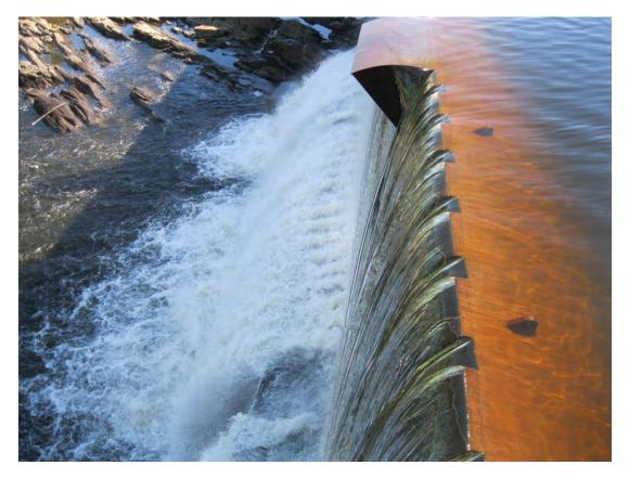
Figure 3-2 Flow conditions at Bascule Gate 1 with 1,500 cfs discharge; note spill jet interaction with concrete sill.
