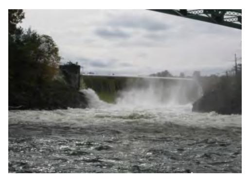
Figure 3-3 Downstream of Bascule Gate 4 at 5,000 cfs.
