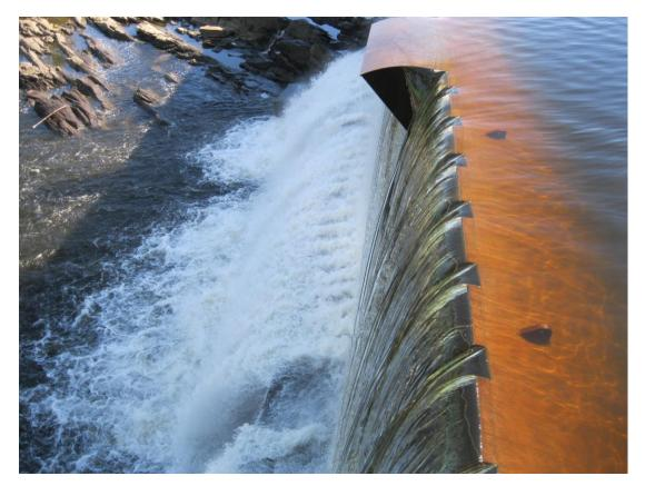
Figure 2-2: Flow conditions at Bascule Gate 1 with 1,500 cfs discharge; note spill jet interaction with concrete sill.
