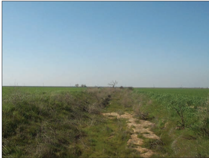
Photograph 3 : Schmidt Creek Ditch.
