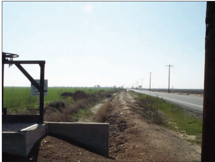
Photograph 4 : Irrigation Ditch control structure.
