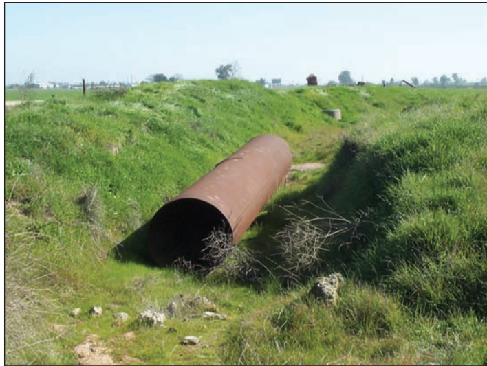
Photograph 2 : Schmidt Creek Ditch.
