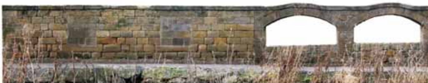
Elevation of the northern section of the east wall of Lesbury Mill. Photo: PCA Ltd
