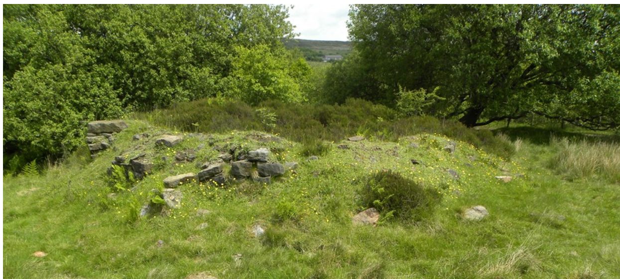
Fig 2c: remains of mine building at Location 6
