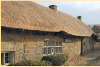
Spout House – simple construction
