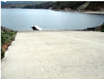
Existing boat launch and dock during draw down
