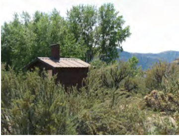
Vault toilet at Keller Ferry
