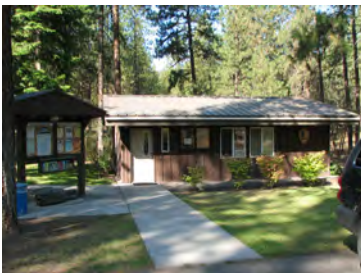
NPS Facilities at Kettle Falls
