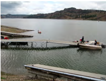
Docking facilities at Porcupine Bay
