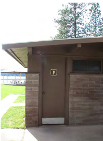
Restroom facility at Evans
