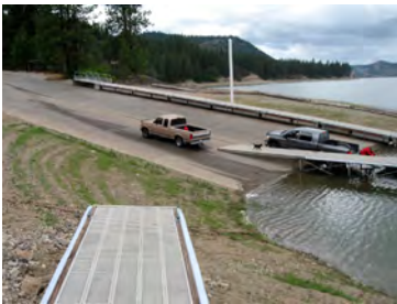
Boat ramp at Porcupine Bay
