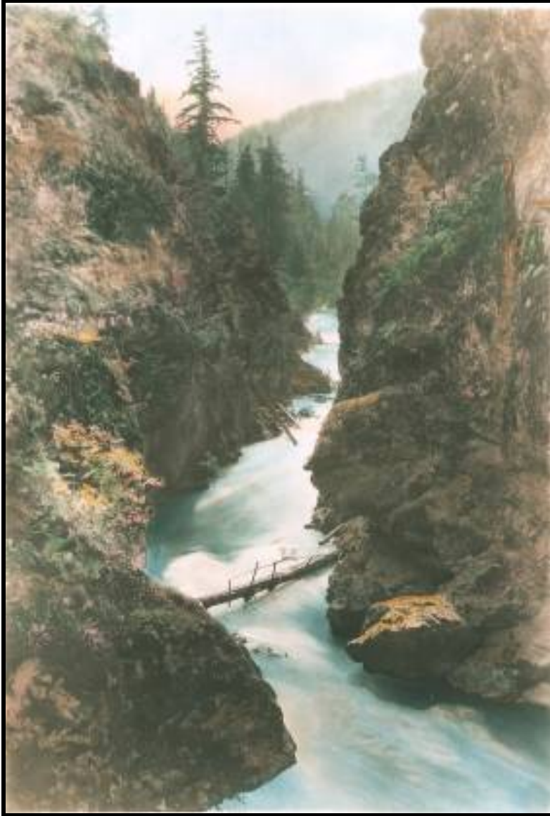
Figure 11. Hand-colored image of black and white photograph showing Glines Canyon and footbridge across Elwha River prior to dam construction, ca. 1900. Courtesy of Olympic National Park. [elwha_07.jpg]
