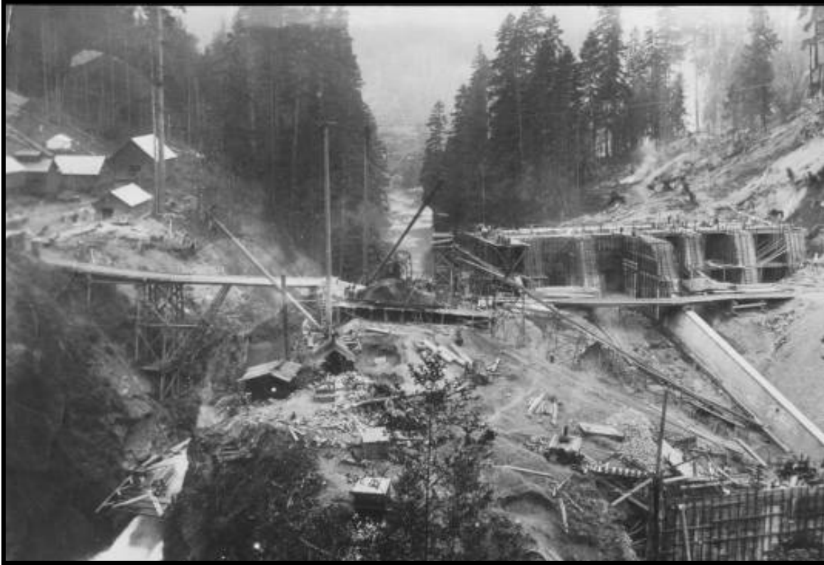
Figure 33. Elwha Dam construction, ca. 1910-1911. Courtesy of Olympic National Park. [Image40.jpg]
