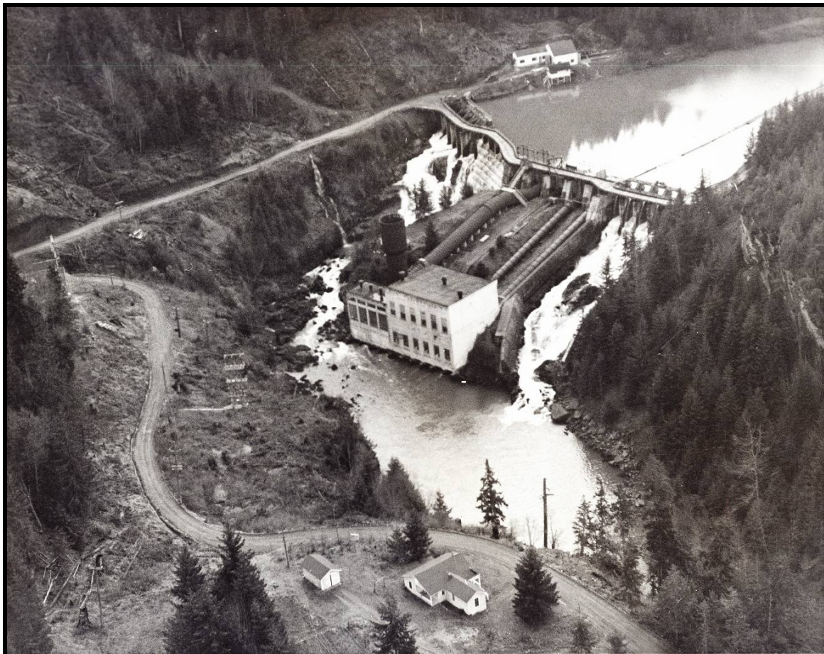
Figure 56. Aerial view of the Elwha Dam, showing power plant annex (left of the main power plant building) and larger-diameter penstock, both added in 1922, n.d. Courtesy of Olympic National Park. [Walsh#8.jpg]
