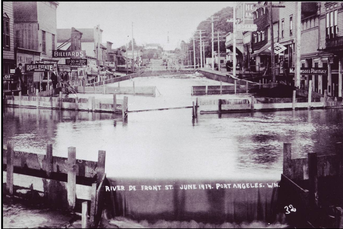
Figure 46. “River de Front,” Front Street in Port Angeles under water during regrade sluicing operations, June 1914. Courtesy of Olympic National Park. [Rotation of PA_RiverdeFront.TIF]
