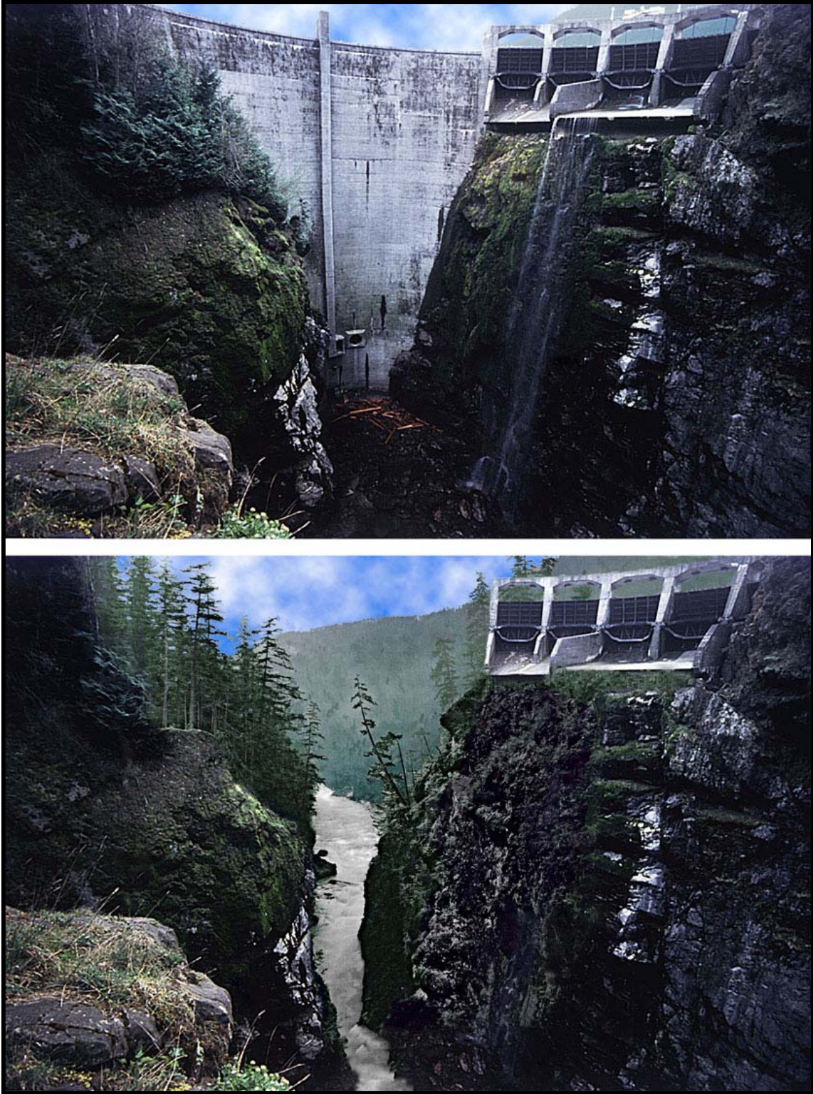
Figure 131. Artistic rendering showing Glines Canyon before (above) and after (below) dam removal. Courtesy of Olympic National Park. [glinestrans_edit.jpg]
