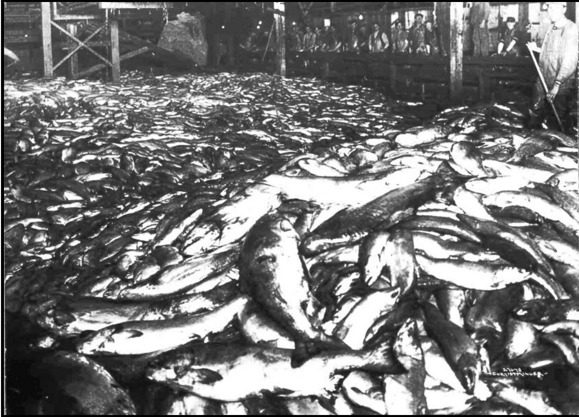
Figure 19. Interior view of cannery. Courtesy of the Bert Kellogg Collection of the North Olympic Library System. [PTAN BLDN – 015.jpg]
