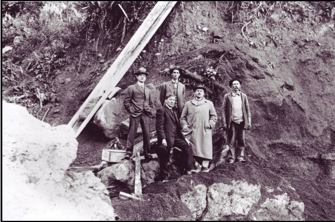
Figure 58. Thomas Aldwell and other company and city leaders at Glines Canyon Dam construction site. Aldwell is the fourth from the left, wearing long overcoat, ca. 1926. Courtesy of Olympic National Park. [HAER_OLYM437_LewisWP&P4.TIF]
