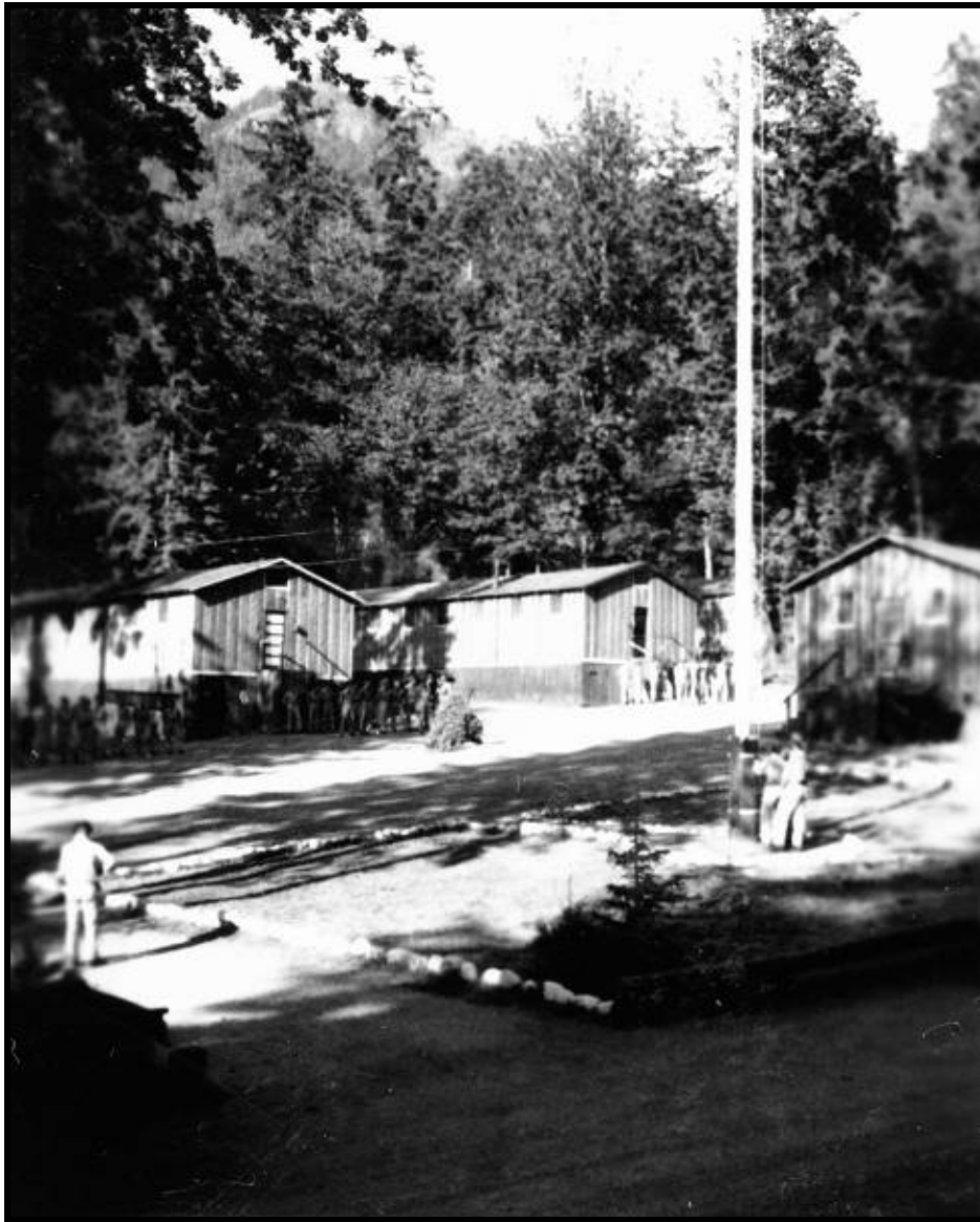
Figure 85. Barracks at Camp Elwha CCC camp. Courtesy of Bernice Byrne. [Byrne_Elwha CC Camp.jpg]
