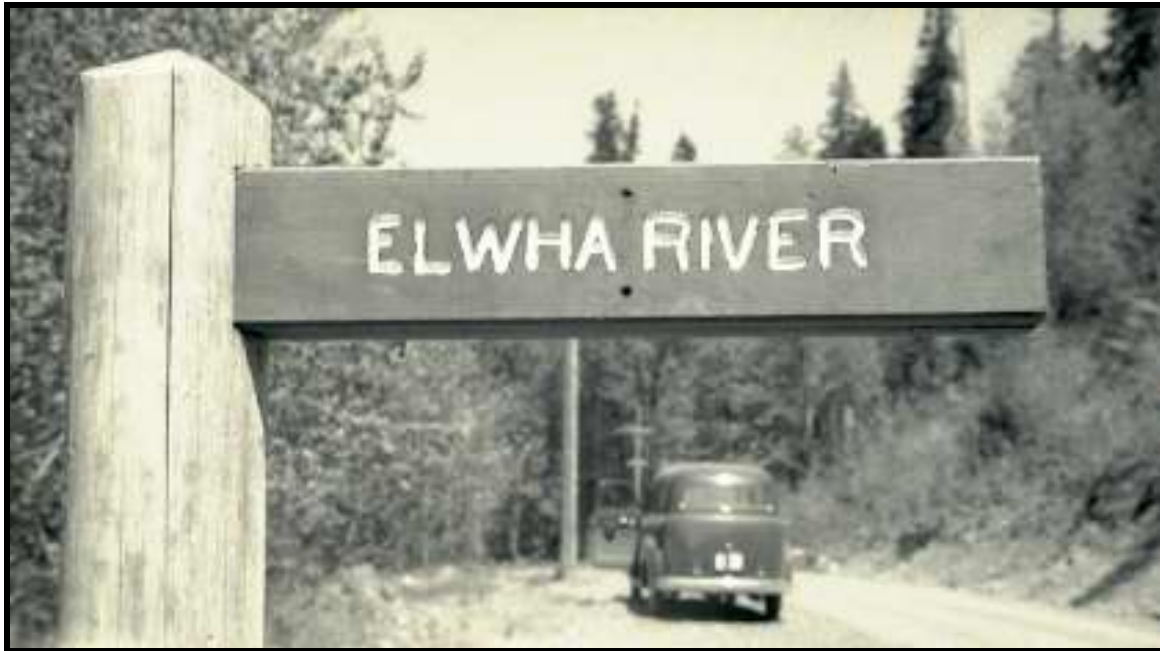
Figure 91. Elwha River sign, 1950. Courtesy of Olympic National Park. [OLYM344783095.JPG]
