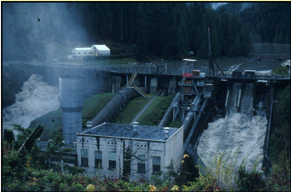
Figure 105. High water flow at the Elwha Dam, n.d. Courtesy of Olympic National Park. [highwaterlwr.jpg]
