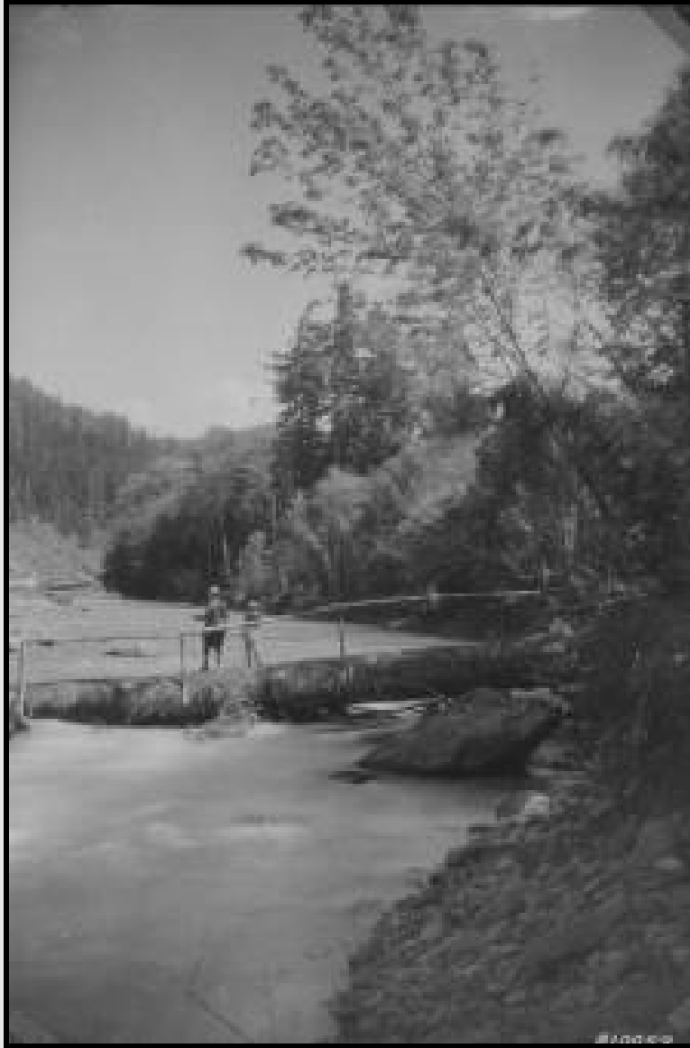
Figure 70. The Elwha River, June 1926. After the Glines Canyon Dam was completed, this spot was 100 feet beneath the surface of the reservoir. USFS photograph. Courtesy of Olympic National Park. [3137_210059.jpg]
