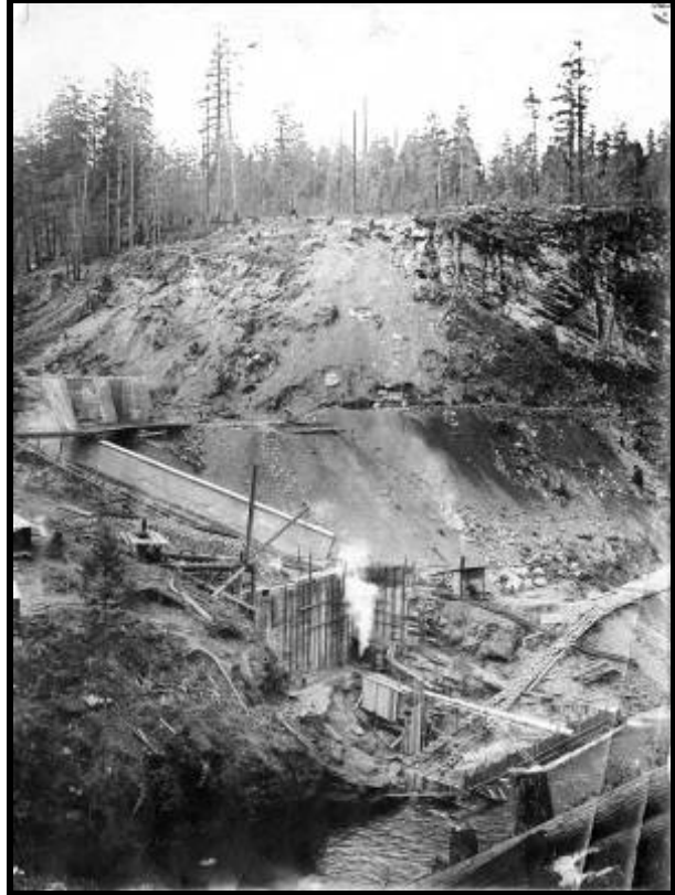
Figure 36. Construction of the powerhouse at the Elwha Dam, ca. 1910-11. Photograph by Critchfield. Courtesy of Clallam County Historical Society, ONP ref. no. 2010.200.147. [2010200147.JPG]
