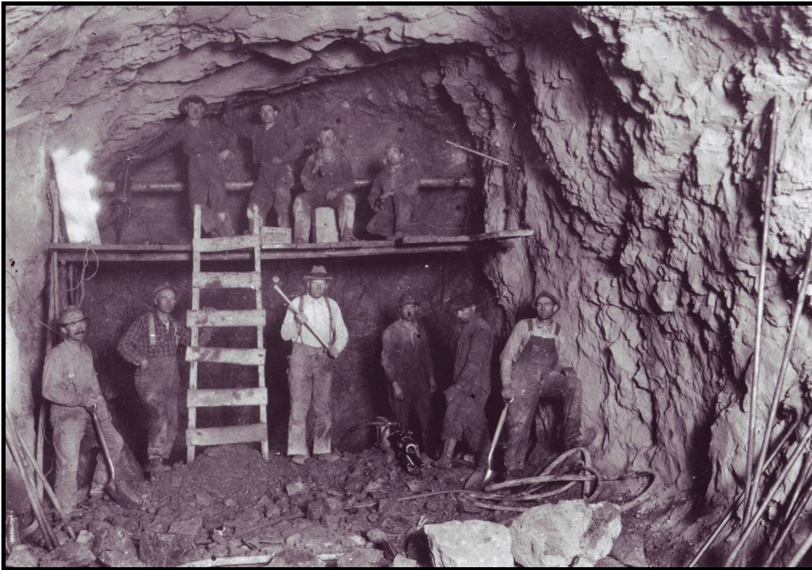
Figure 60. Crew digging bypass tunnel at Glines Canyon Dam, ca. 1926-1927. Courtesy of Olympic National Park. [HAER_OLYM437_Oliver1.TIF]
