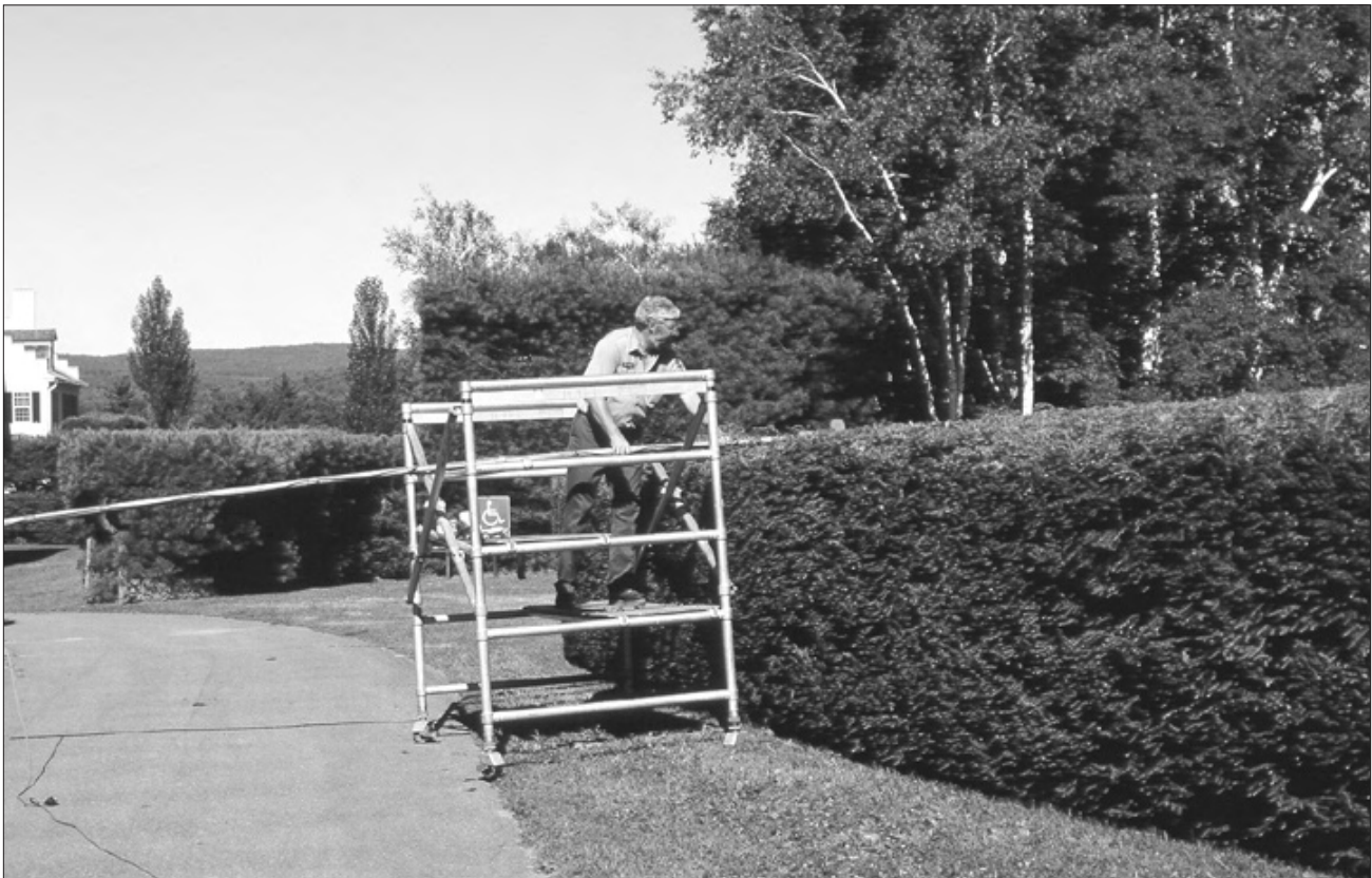
Figure 7. Hedge trimming on scaffolding north of the Caretaker's Cottage (OCLP, 1993).
