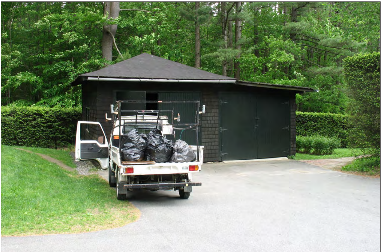
Figure 41. View south of the Caretaker's Garage and driveway with the brick path to the Caretaker's Cottage back door at right and small bed of perennials. Mature pines and the hedge along Saint Gaudens Road are visible in the background (OCLP, 2009).
