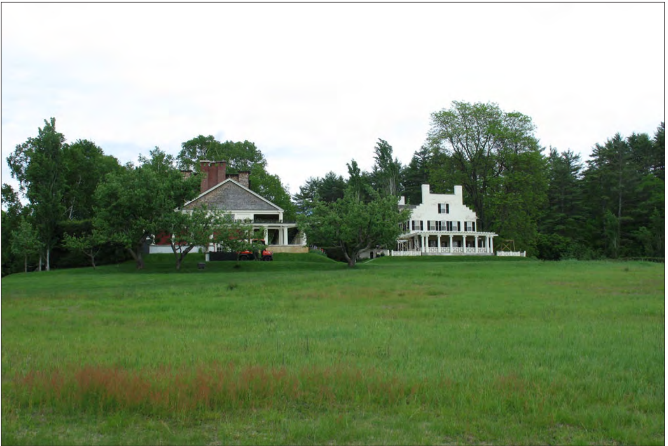
Figure 12. View east of the main house and Little Studio with the west meadow in the foreground. A row of apple trees partially obscures the Little Studio (OCLP, 2009).
