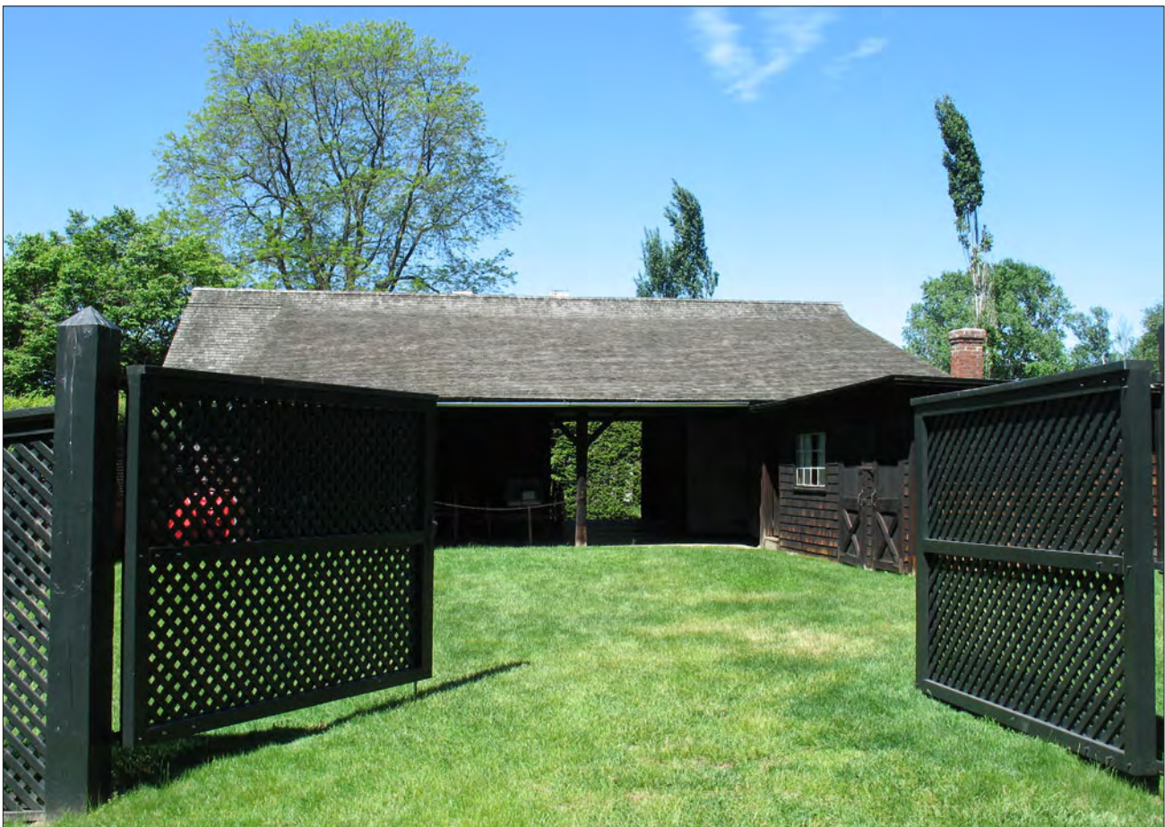
Figure 35. View west of the stables, fence and gate along the east entry drive. The enormous honeylocust in front of the house and tall poplars behind the house and in the gardens are visible in the distance (OCLP, 2009).
