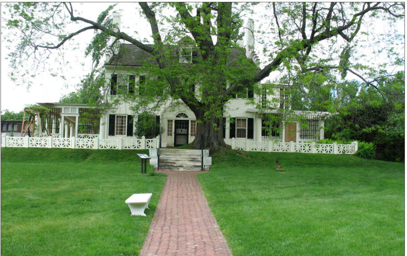
Figure 17. View north of the main house brick walk, bench, marble steps, park wayside, and terrace balustrade. A bed of roses and ferns is partially visible by the southeast corner of the house behind the balustrade at the far right. The mature honeylocust obscures the house facade (OCLP, 2009).
