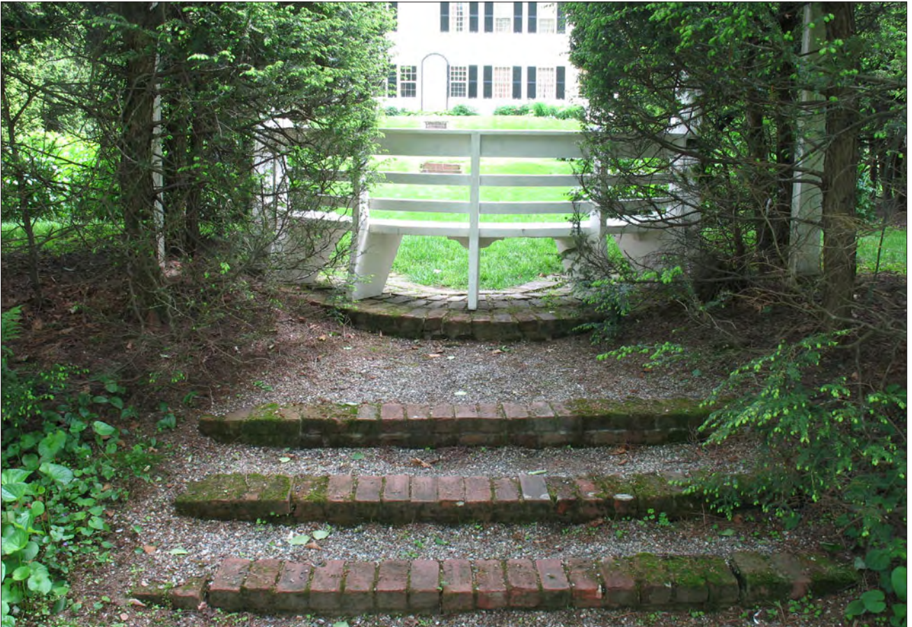
Figure 29. View south of brick steps and hedge opening between the flower garden and birch allée, now blocked by bench (OCLP, 2009).
