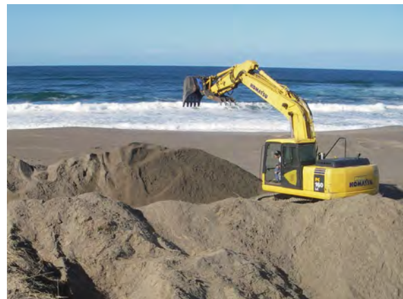
Excavator moves sand to bury European beachgrass.
