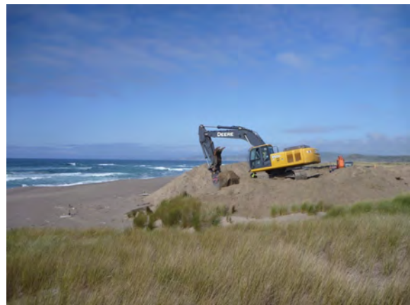
Excavator removing European beachgrass
