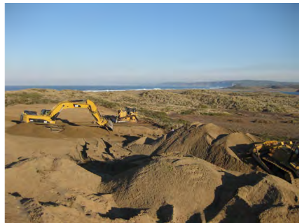
Excavators with mounds of sand for horizontal flipping
