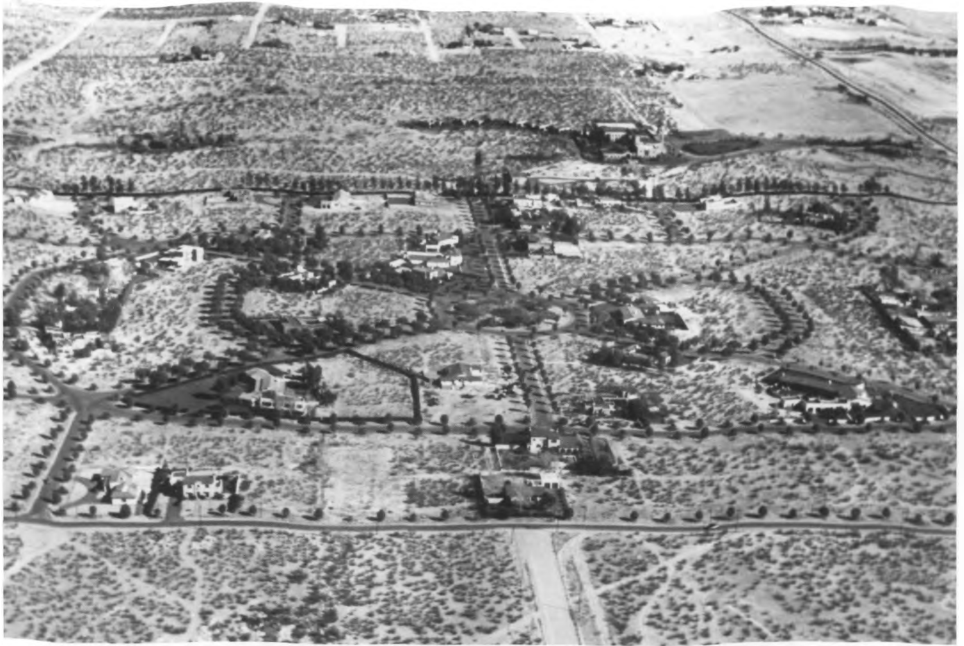
An oasis in the desert, Tucson's El Encanto Estates evolved from a geometrically perfect radial plan (1929) designed in the office of a California engineering firm and later laid out by field engineers on the floor of the Sonoran desert. A c. 1934 aerial photograph (above) depicts early improvements, including the layout of streets and spacious lots, rows of evenly-spaced street trees, and a central, circular park. A sales map (left) prepared in 1951 indicates the extent to which streets had been extended and lots further subdivided following World War II. Supplementing State survey forms, a horticultural inventory form was used to record information about the Mexican fan palms ( Washingtonia robusta ) and date palms ( Phoenix dactylifera ) lining the streets and the stately collection of giant saquaro ( Carnegiea gigantea ) gracing the central park. (Photo and sales map courtesy Arizona Historical Society Library/Tucson)
