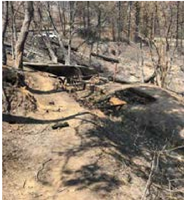
Crystal Creek Clean-out Shed remnants and mechanical system, looking east, 8/15/18.
