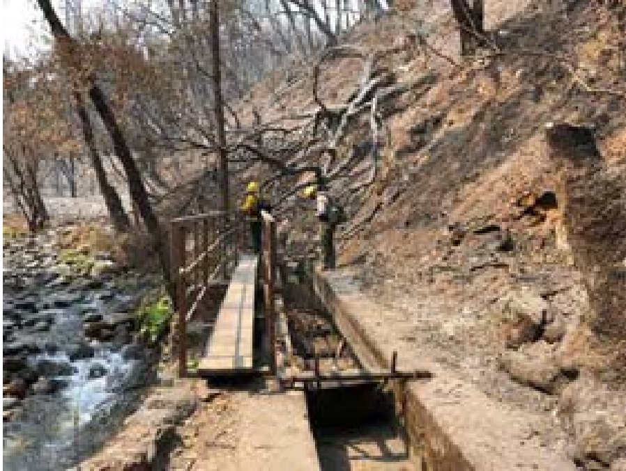
Crystal Creek overflow and sluice, looking west, 8/21/18.
