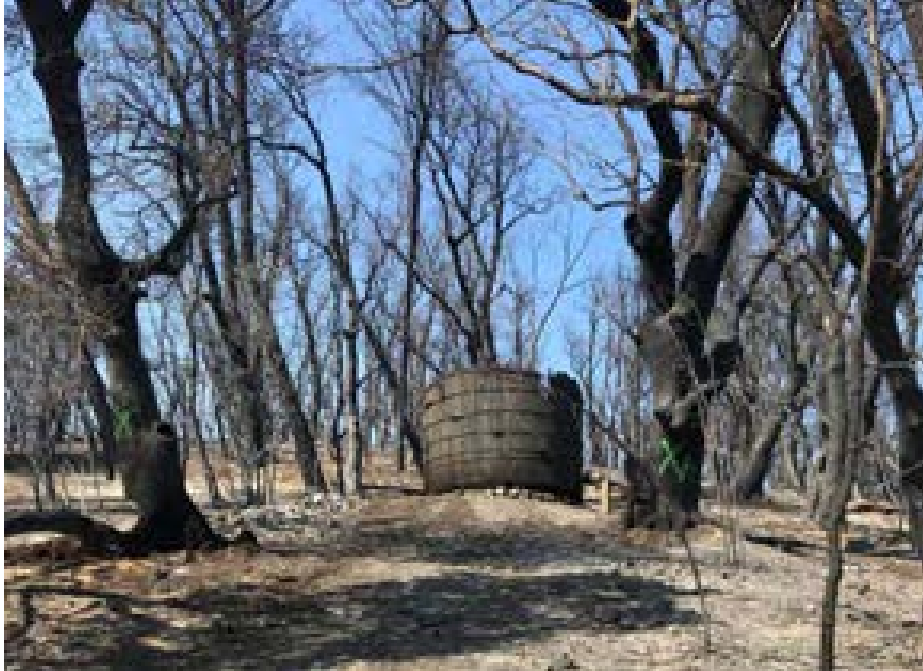
Crystal Creek Water Storage Tank, looking north, 8/15/18.
