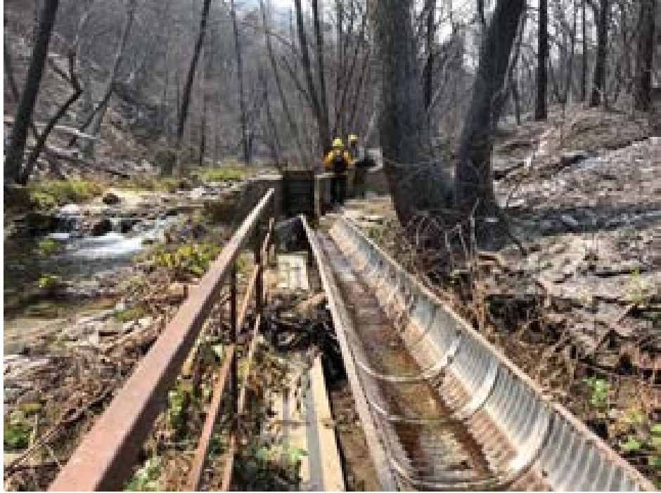
Crystal Creek Ditch intake and flume, looking west, 8/21/18
