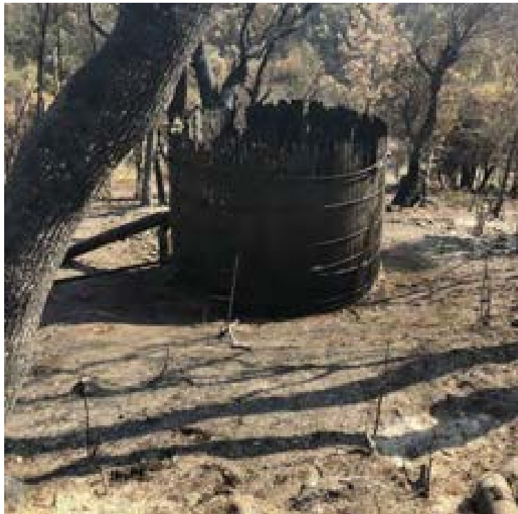
Crystal Creek Storage Tank, looking south, 8/15/18.
