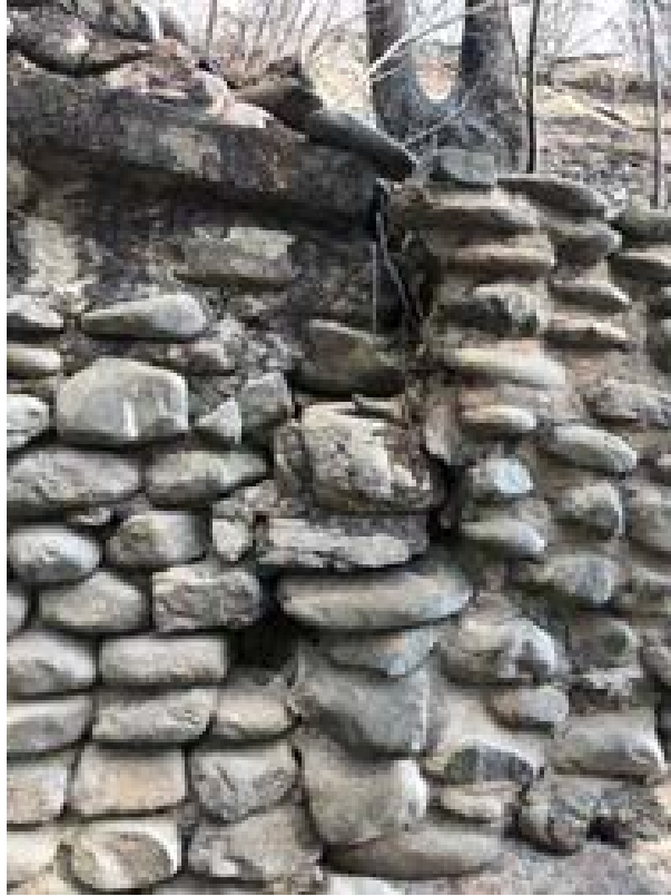
Stone House, Retaining wall, 8/16/18.
