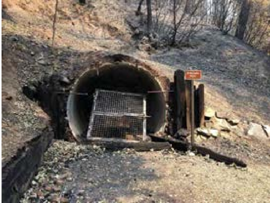
El Dorado, primary mine opening, looking north, 8/14/18.
