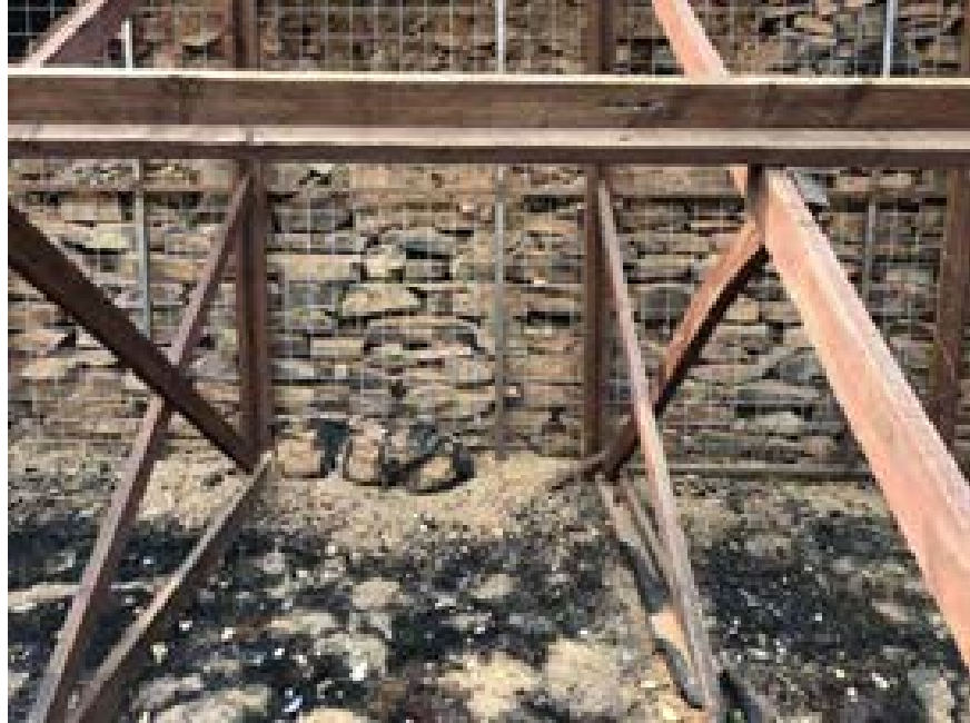
Blacksmith Shop back wall, looking north, 8/14/2018.
