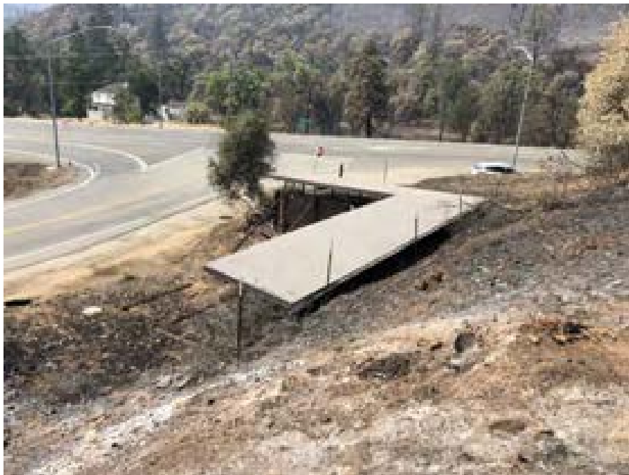
Blacksmith Shop, looking south, 8/14/2018.
