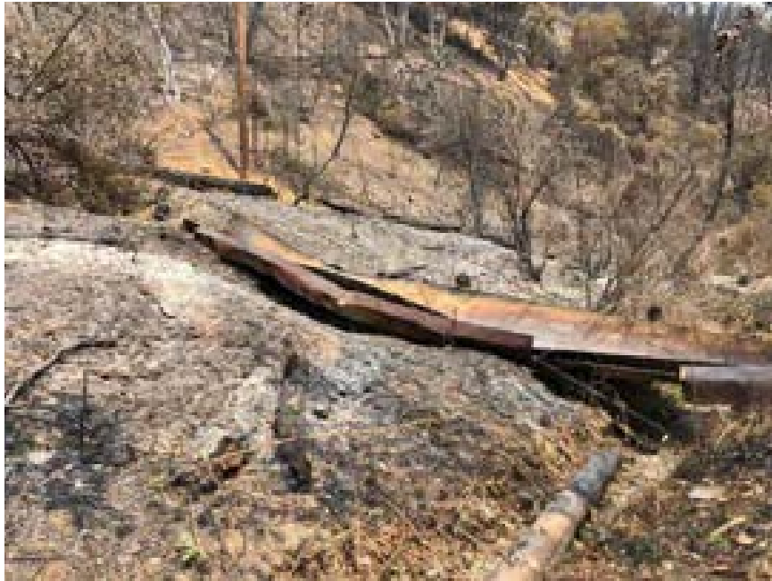
Crystal Creek Ditch culvert, looking northwest, 8/21/18.
