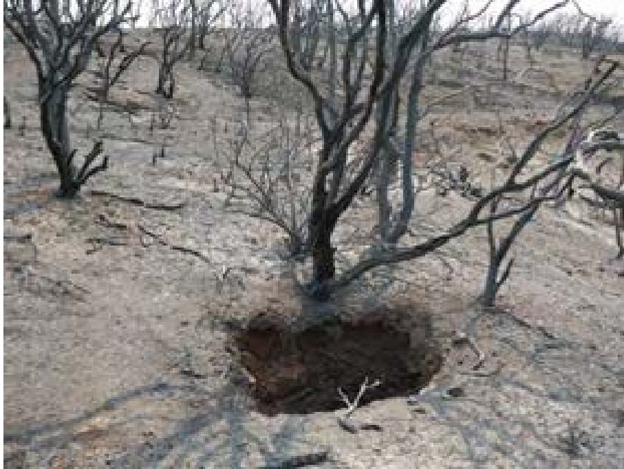
Open vertical shaft along West Side Trails
