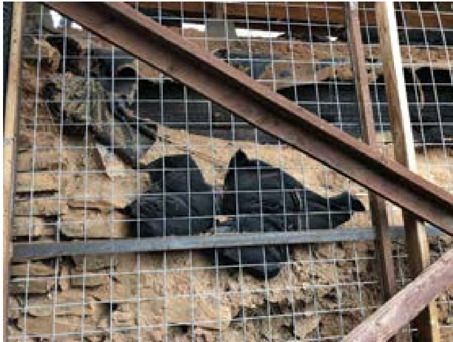
Blacksmith Shop back (north) wall. Image shows burned cribbing and fallen sandbags, 8/14/18.
