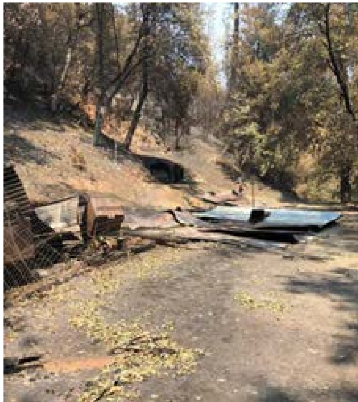
El Dorado mine entrance and building remnants, looking northwest, 8/14/18.
