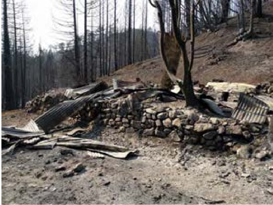
Burned structure at Brown Bear Mine
