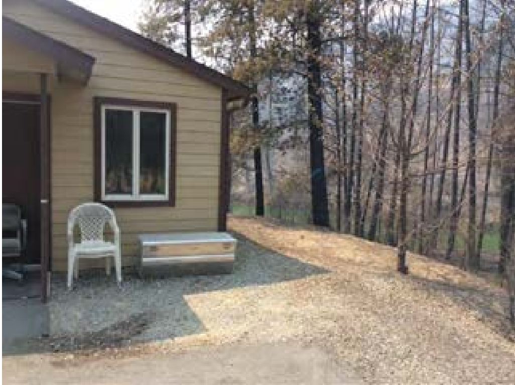
Hazard Tree at Water Treatment Site
