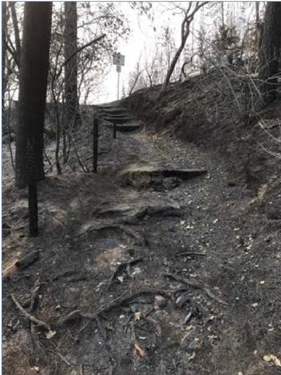
Burned stair treads and handrail.
