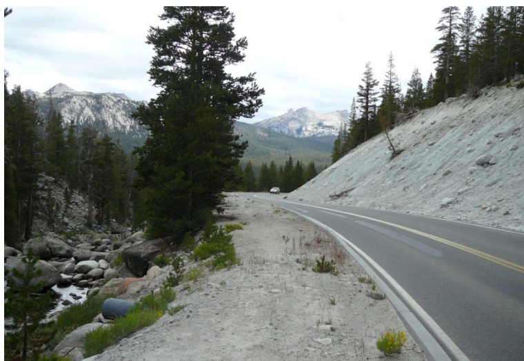
Fine soils along a portion of Tioga Road can contribute to river turbidity during storm events.
