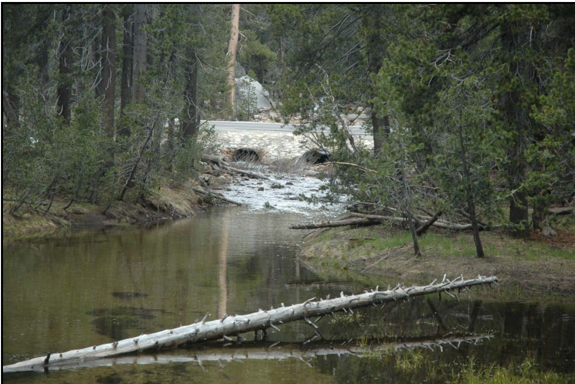
Photo D- 8. Murphy Creek Culverts under Tioga Road
