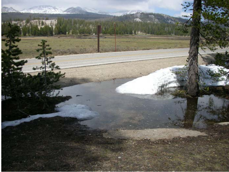
Figure 2-18. Ponding observed upstream of road, near Transect 2 and Budd Creek.
