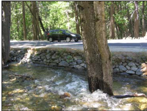
Seasonal flooding at Bridalveil Creek drainage
