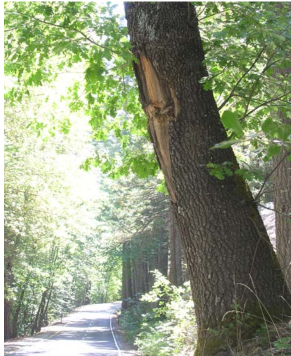
Figure III-6. Large oak tree leaning over the Yosemite Valley Loop Roadway that has been damaged by plows and large trucks. (NPS Photo)
