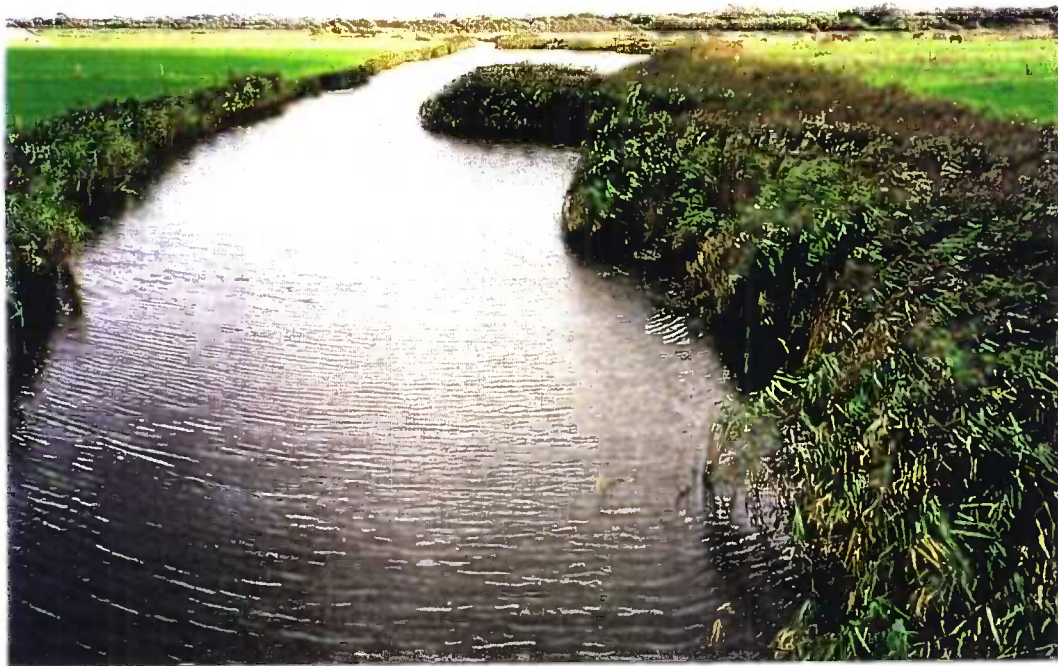
Plate 4.1.6 View of channel running under the road bridge (Sta. 5). Ballyteige drainage channels, Co. Wexford. 1998.
