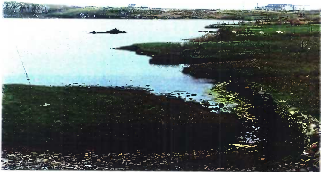
Plate 4.11.2 View of northwest corner of the lagoon showing seepage through the barrier (Sta. 1). Lough Bofin, Inishbofin, Co. Galway. 1998.
