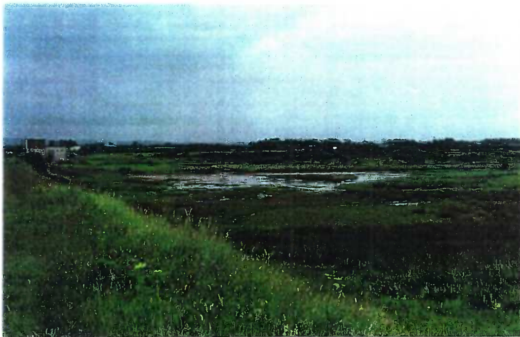
Plate 4.1.2 View looking north along sea wall towards pumping station. Ballyteige drainage channels, Co. Wexford. 1998.
