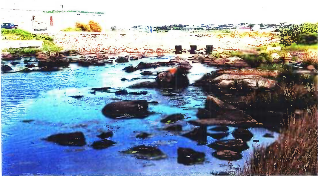
Plate 4.15.1 View of bridge and sluices at the north end of the lough. ( Sta. 1). Moorlagh, The Rosses, Co. Donegal. 1998.
