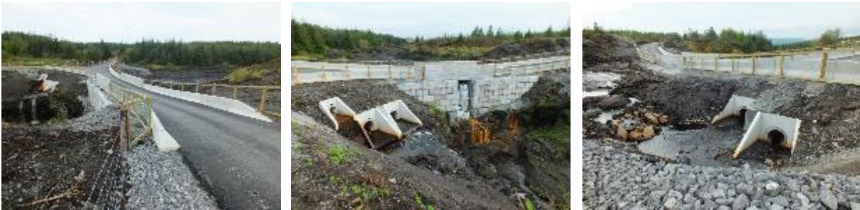
Figure 8-1 Completed Remedial Works at the Dawn of Hope Bridge
