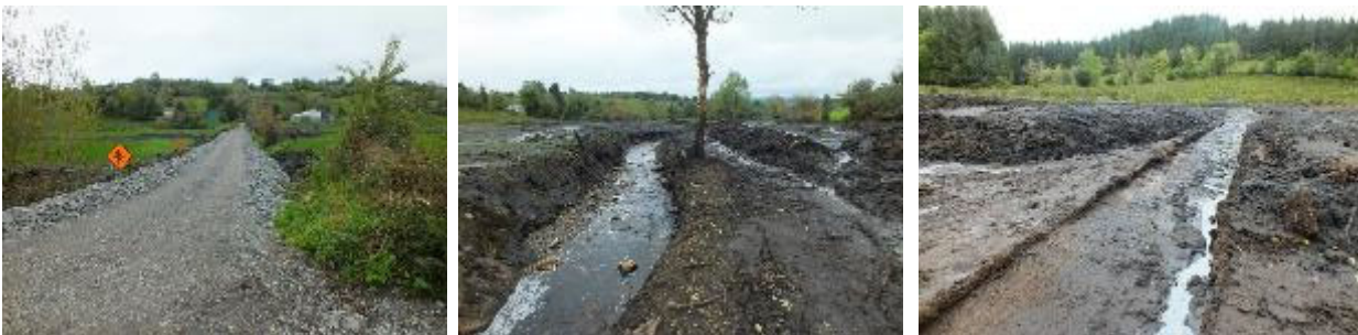
Figure 8-2 Completed Remedial Works at Corcormick
