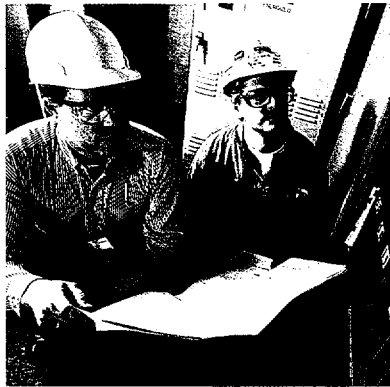
Above: Jim Martin (left) and Mark Green examine a battery rack improvement made at the Belle River Power Plant.
