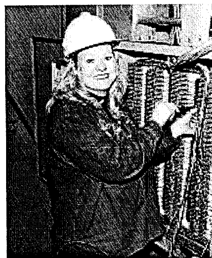
Apprentice Electrician Peggy Jenschke helps with substation construction and maintenance.
