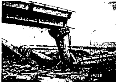
Figure 15 : Failure due to longitudinal Slip, Taiwan 1999
