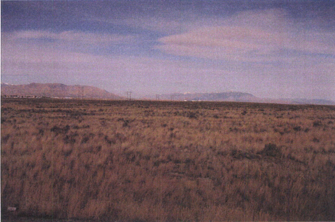
Figure H-5e. Transmission lines on the west end of the transmission corridor leading to the Antelope Substation, facing northwest.
