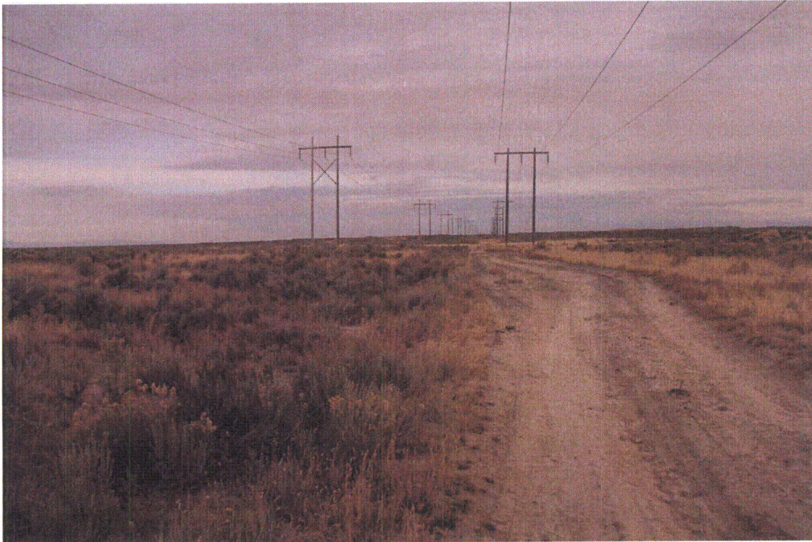
Figure H-5f. Existing transmission lines along two-track road on the east end of the transmission corridor between the Bonneville Substation and U.S. Highway 20, facing north.
